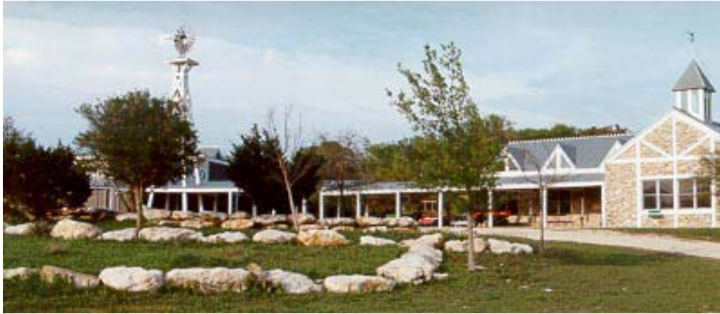
Figure 1: Camp John Marc, Dining Hall and Saddle Room
