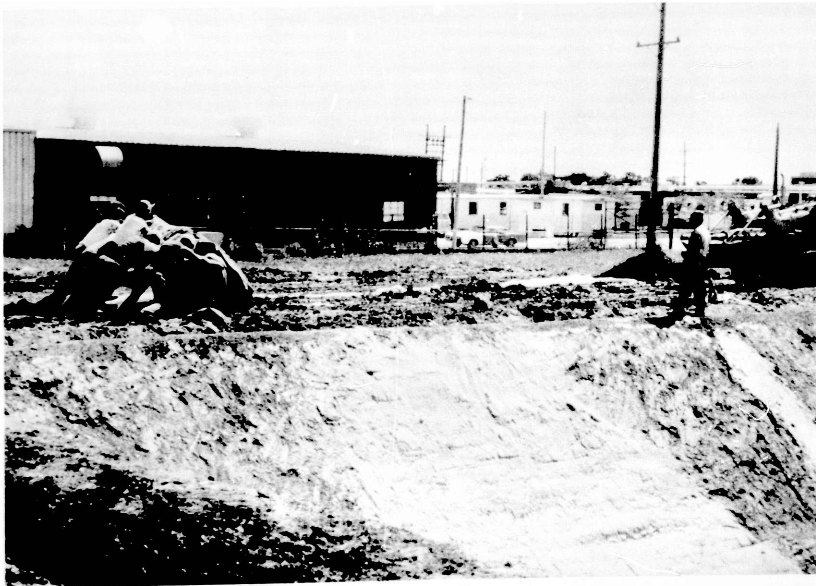
Fig. 15. Unfolding the Liner on the West Bank of the Pond
