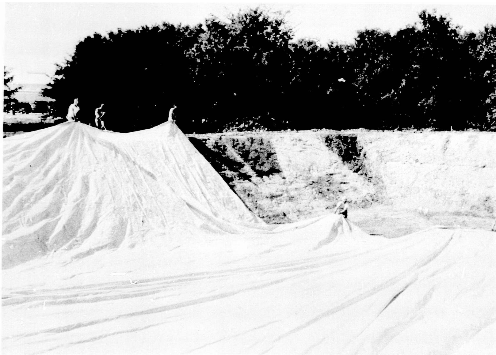
Fig. 19. Two-thirds of the Pond Covered with the Liner
