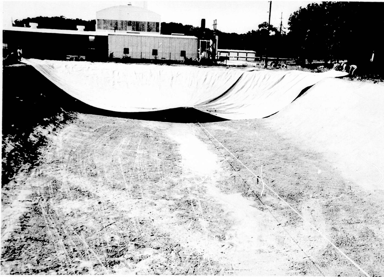
Fig. 18. Another View of Liner Unfolding
