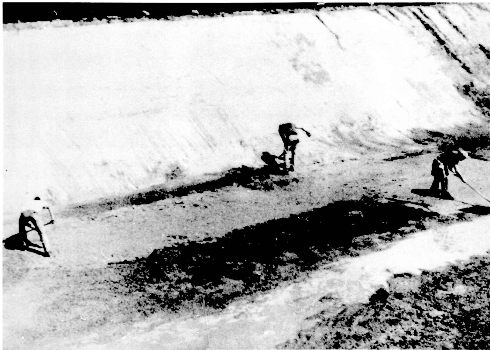
Fig. 14. Sand Application at the Bottom of the Pond
