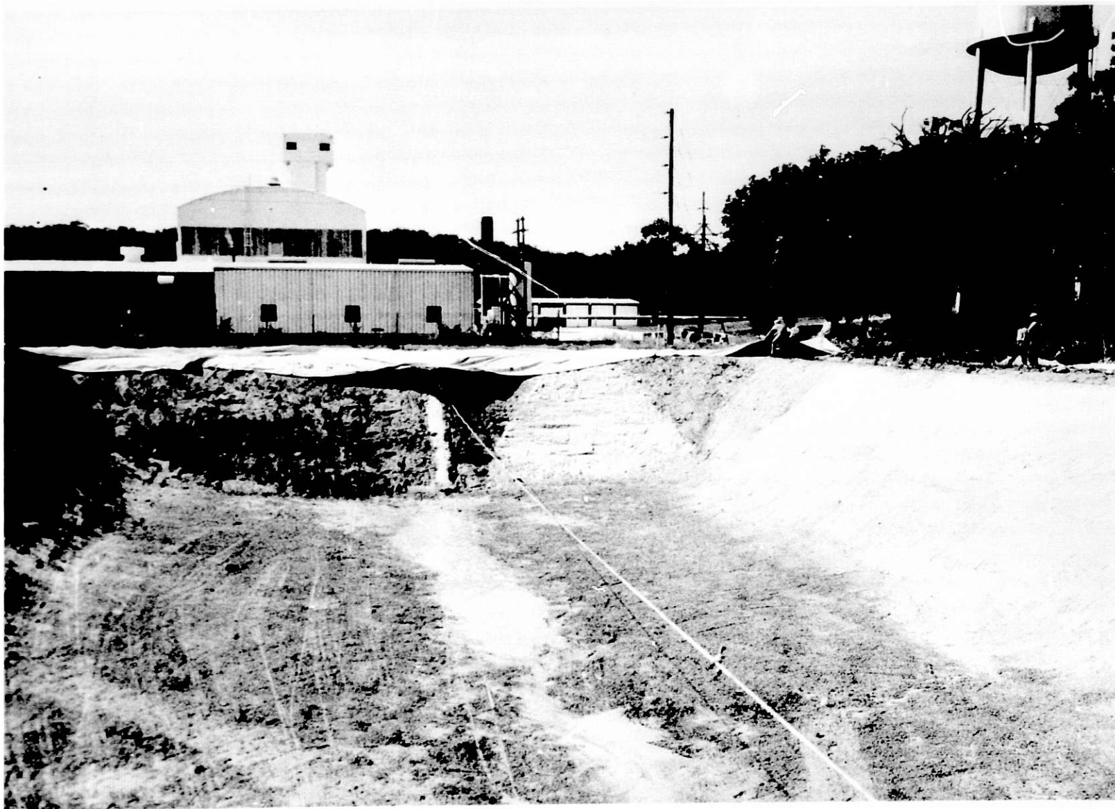
Fig. 17. Front-end Loader Beginning to Pull the Liner Across the Pond
