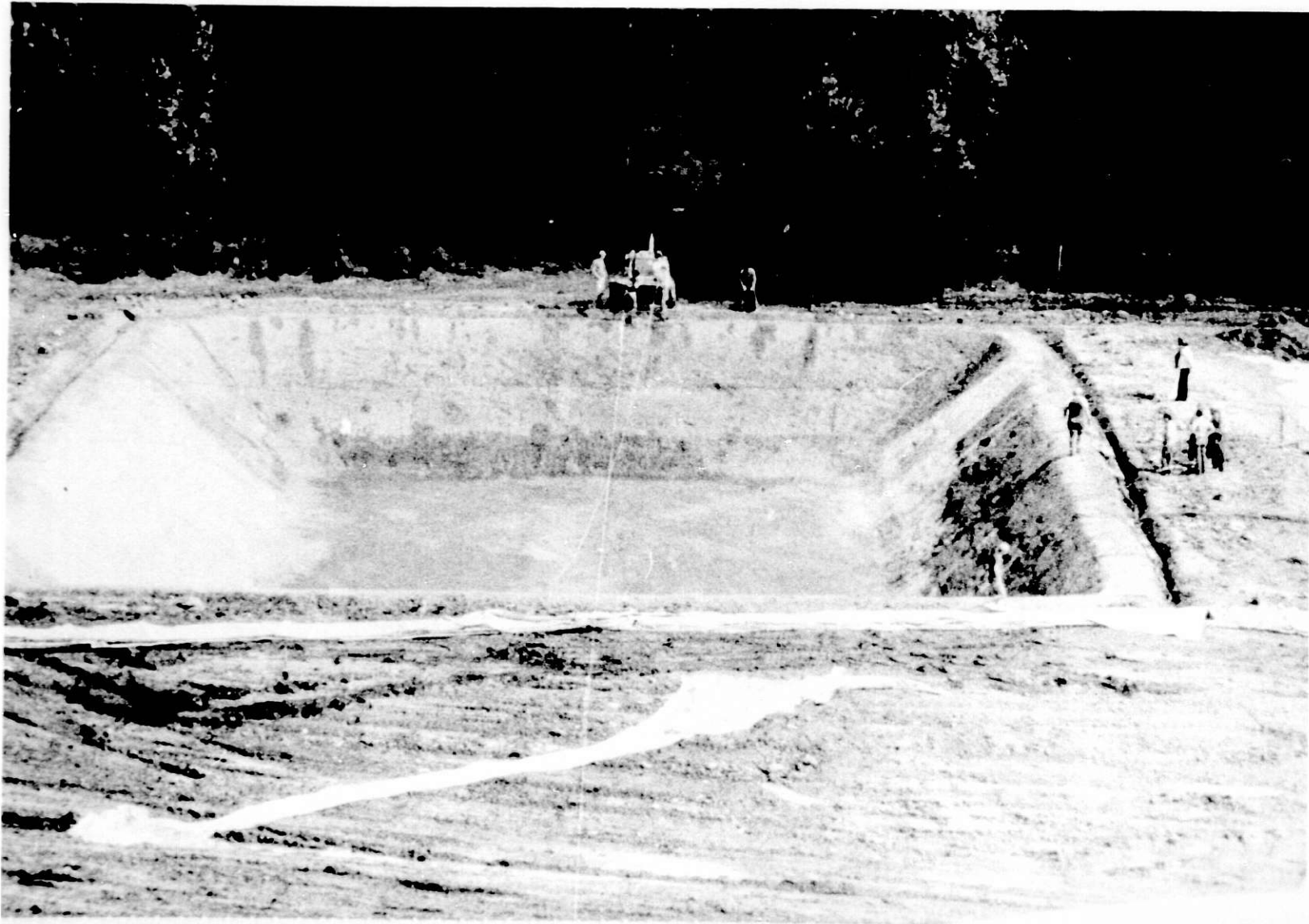
Fig. 16. Liner Ready to Be Unfolded Across the Pond
