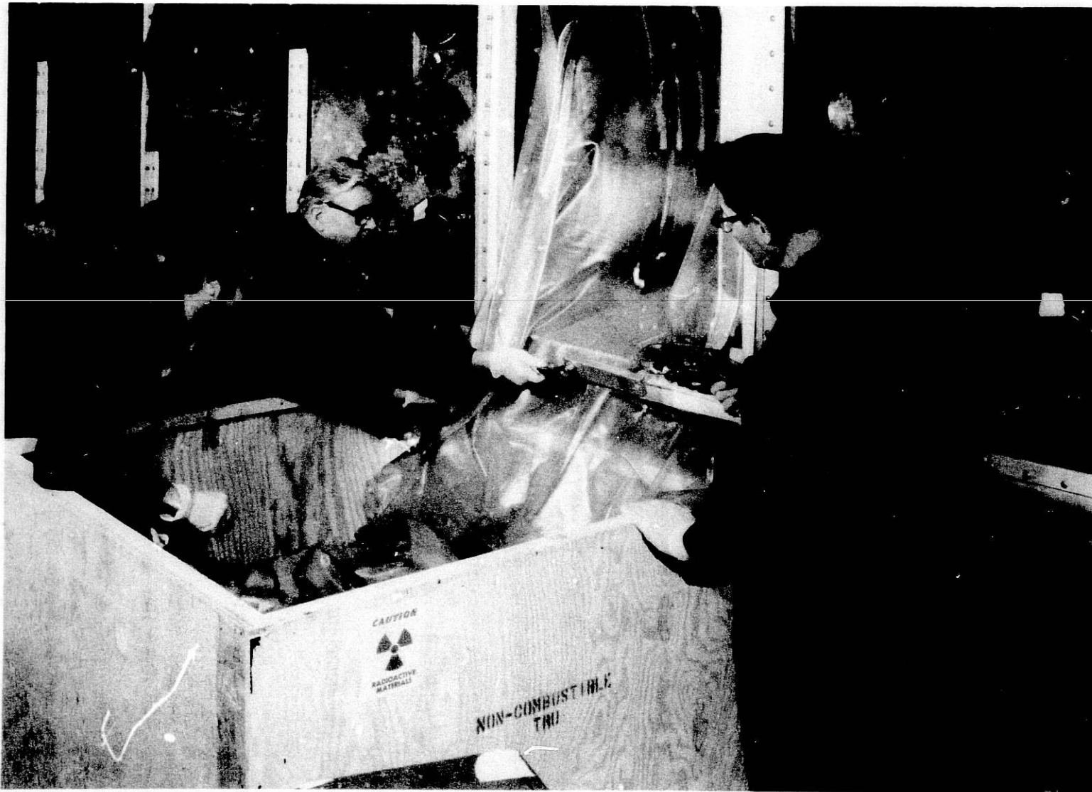
Figure 4-12 Sealing Bagout Pouch Filled with Waste
