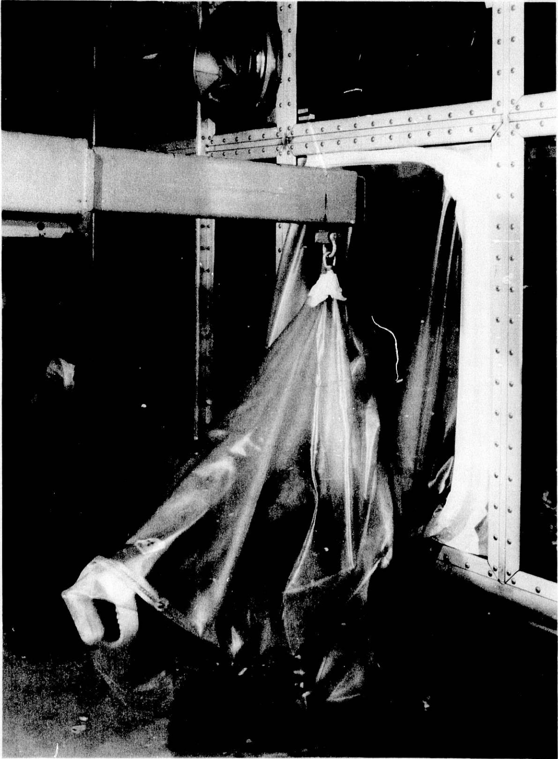
Figure 4-13 Waste Removal Assisted by a Fork Truck Boom
