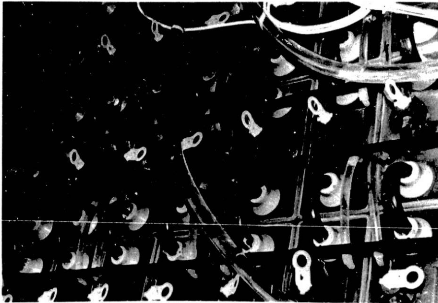
Fig. 7: VARTA watering and degassing system
