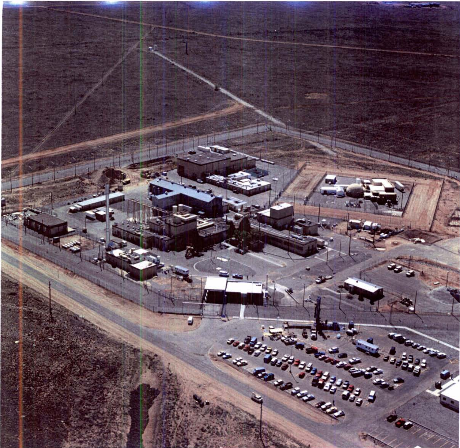
Tech Area V - Northwest
