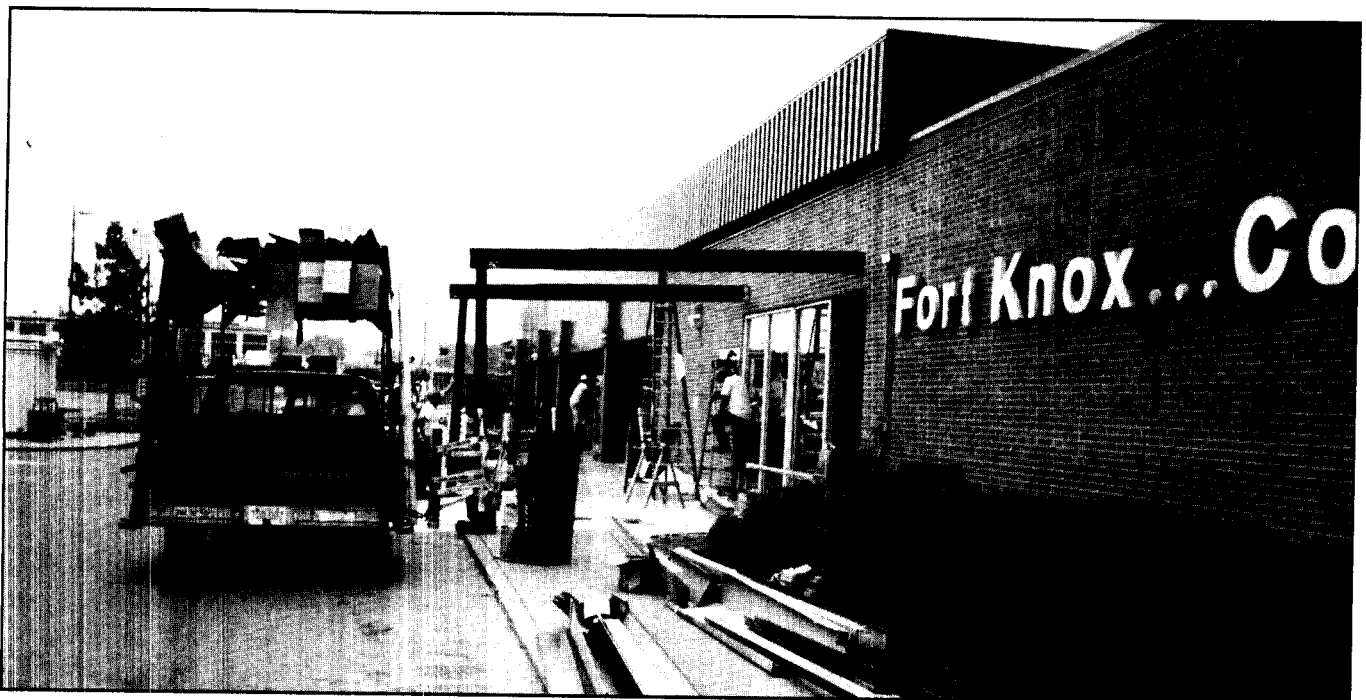
The contractor coordinated his schedule with the store manager on a weekly basis to minimize inconveniences to shoppers. Here, work progresses while the store is closed.
