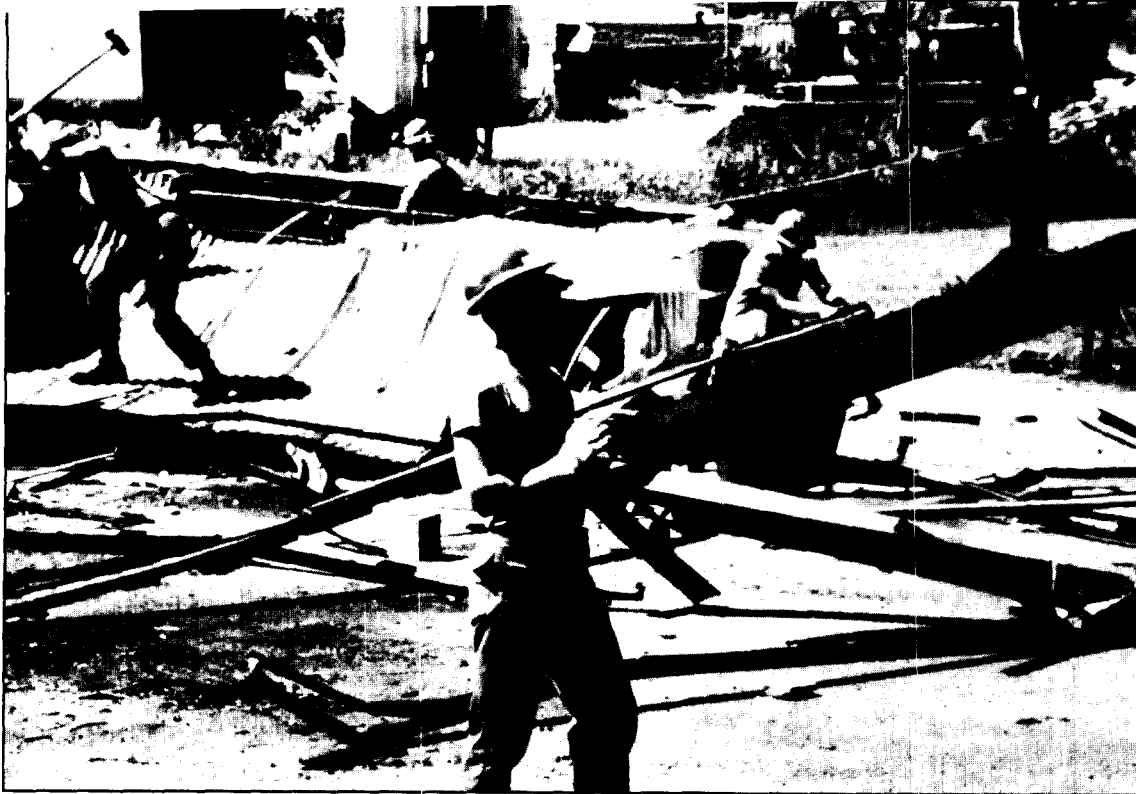
Nearly 800 Seabees were involved in recovery efforts in the wake of Hurricane Andrew. Here, they are cleaning up a neighborhood in Dade County, Florida.
