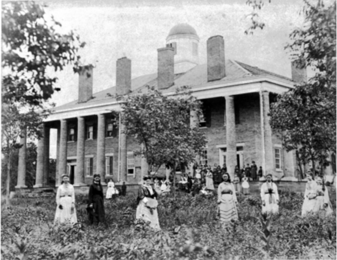
12. Graduating class of 1875 of the young ladies seminary near Tahlequah. Building cost $45,000. Erected by the Tribe in 1857, with their own money and supported by them. John K. Hillers, 1875. Archives and Manuscripts Division of the Oklahoma Historical Society.
