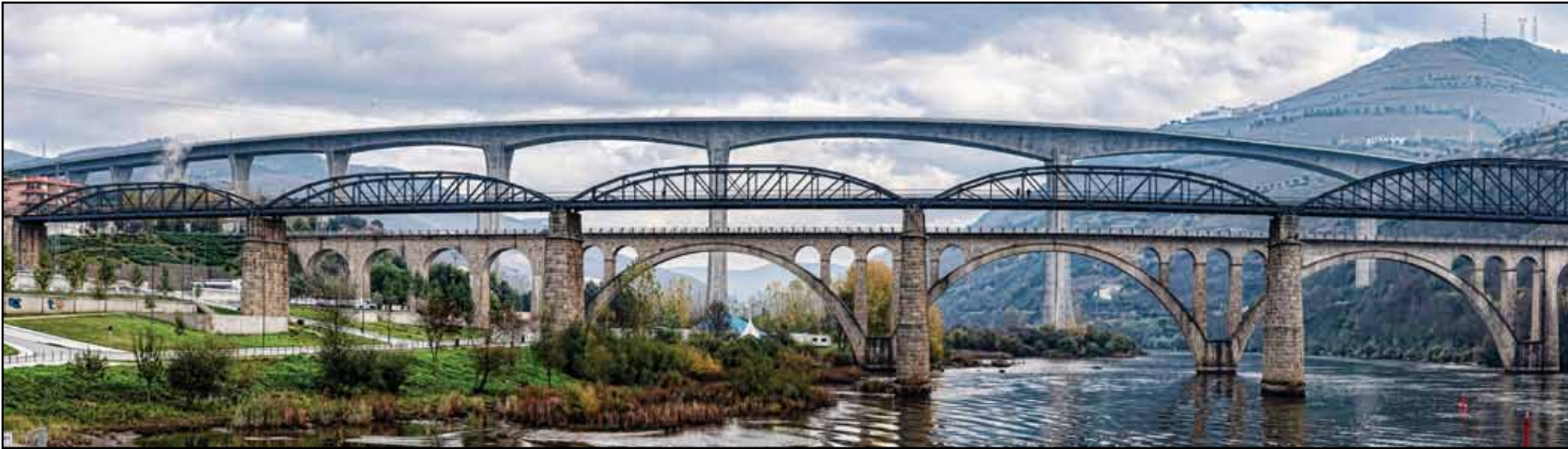
Douro River Bridges, Portugal. By Tom Sheckels.
