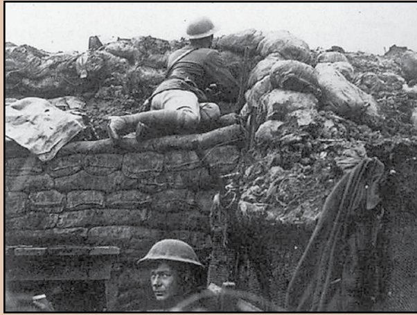
OGS Crawford in Trench (foreground).
