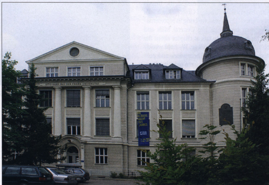
Figure 2. The Kaiser Wilhelm Institute is now the Freie Institute, located in Berlin-Dahlem, Thielallee 63—N52° 26.85 E13° 17.11. This is the Hahn-Meitner-Bau (Building): Institut für Biochemie, the laboratory where the splitting of the atom was first observed.
