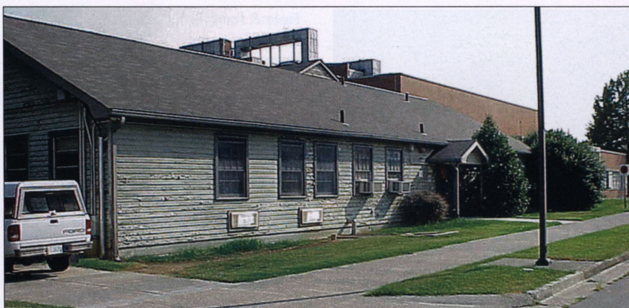
Figure 9. Chemical Analysis Building, Oak Ridge, TN, where promethium was isolated (originally the west wing of the building complex; then building #706, now building #3550, Central Ave.—N35° 55.61 W84° 18.99). The actual laboratory where the separation of promethium was done is at the far end, where now a modern brick building stands (visible behind the wooden structure).
