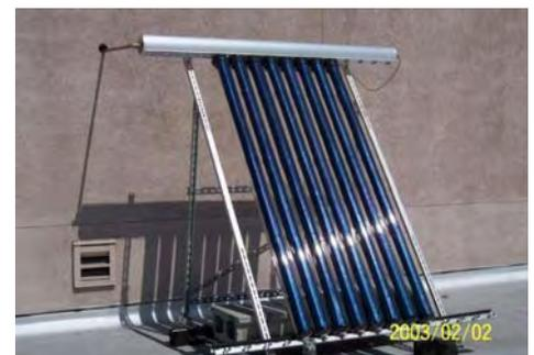
*Photo 4: A Solar thermal water heating system installed by staff at Yakima Valley College.*
