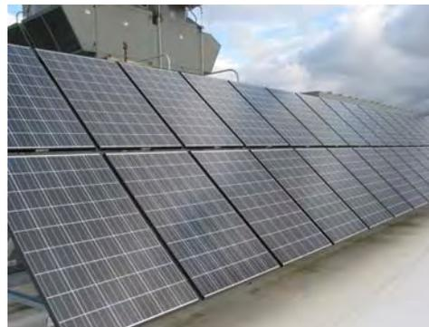
*Photo 6: In the past year, Skagit Valley College has generated nearly 36,000 kwh from a Solar photovoltaic array on top of LEED Platinum Laura Angst Hall.*
