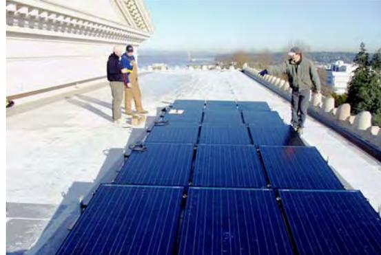
*Photo 11: GA installed solar panels with the help of Puget Sound Energy. GA uses the panels to power the lights at the top of the dome of the*
