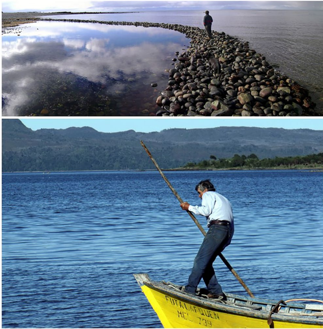
Figure 7. (top) A fishing weir on Caguach Island, Chiloe archipelago. This stone dam is traditionally built to catch fish taking advantage of the cycle of the tides, the moon, and the seasonal migrations of fish. (bottom). Local fisherman on his boat in the Guaitecas archipelago south of Chiloe (Photographs Ricardo Álvarez, 2008).
