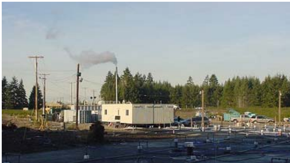
Thermal Remediation, Fort Lewis Log Center, Feb 2004
