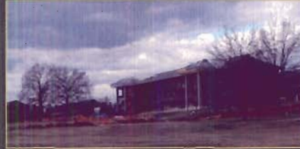
$3.5M Renovation of Permanent Party Dormitory
