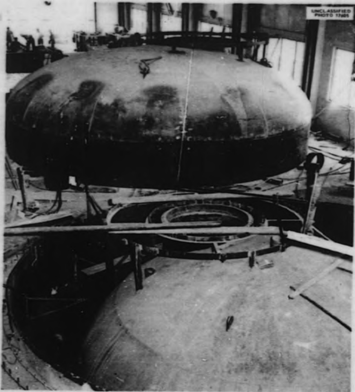
Fig. 1.5.3. Pressure Vessel and Water Tank That Make Up the Reactor Cell. Photograph taken May 11, 1956.
