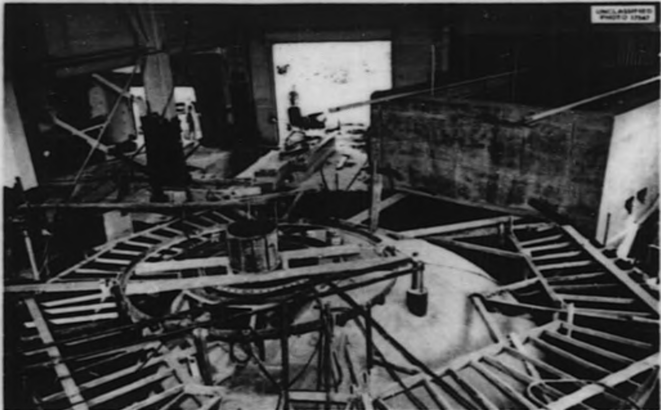
Fig. 1.5.4. Concrete Penthouse Adjacent to Reactor Cell. Photograph taken May 4, 1956.
