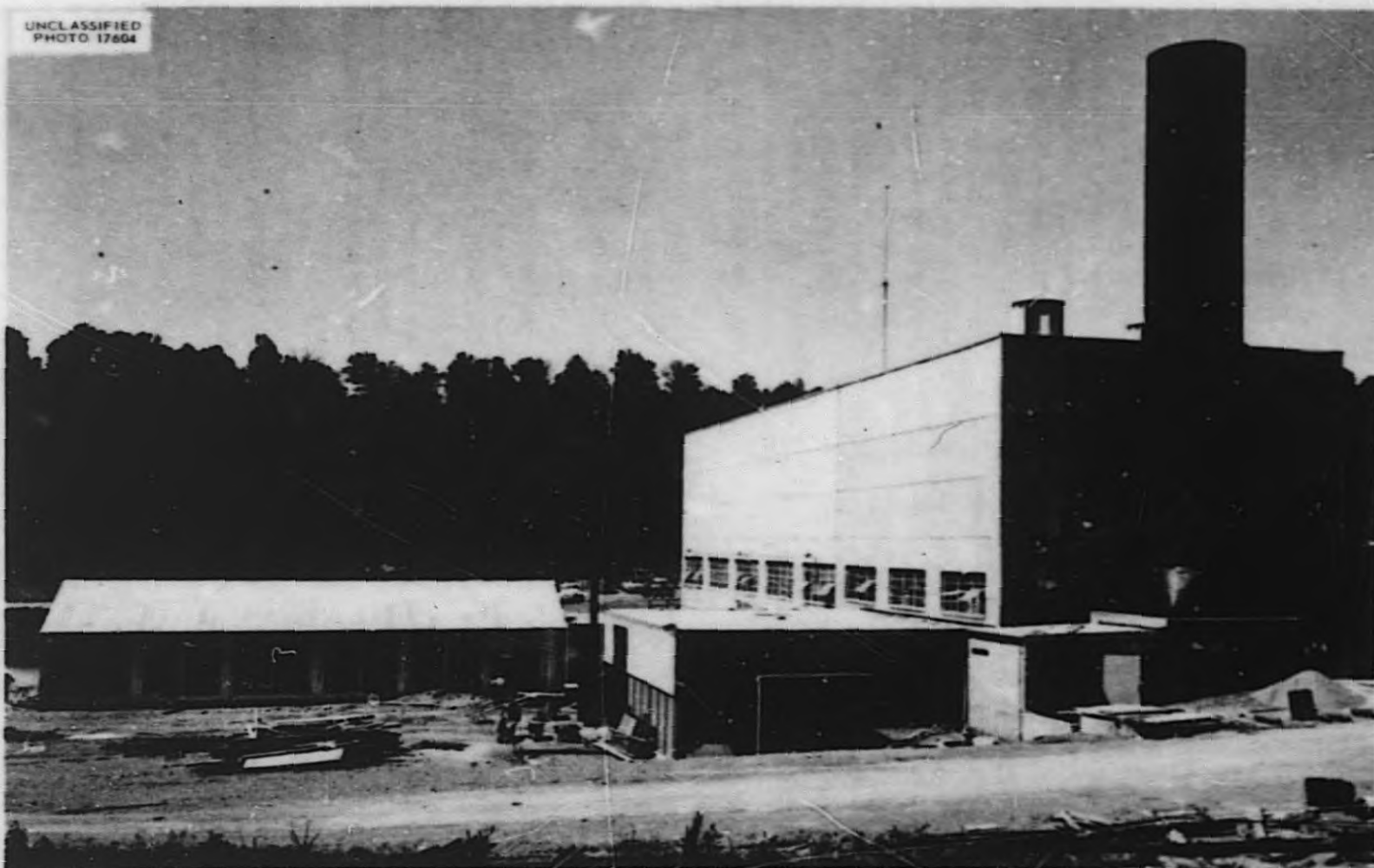
Fig. 1.5.1. View of ART Facility Building 7503 from a Location Southwest of the Building. Photograph taken May 11, 1956.
