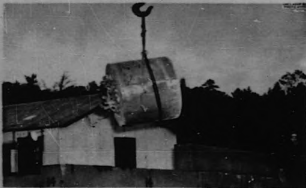
Fig. 21. Reactor Being Removed from Storage for Transfer to Burial Ground.
