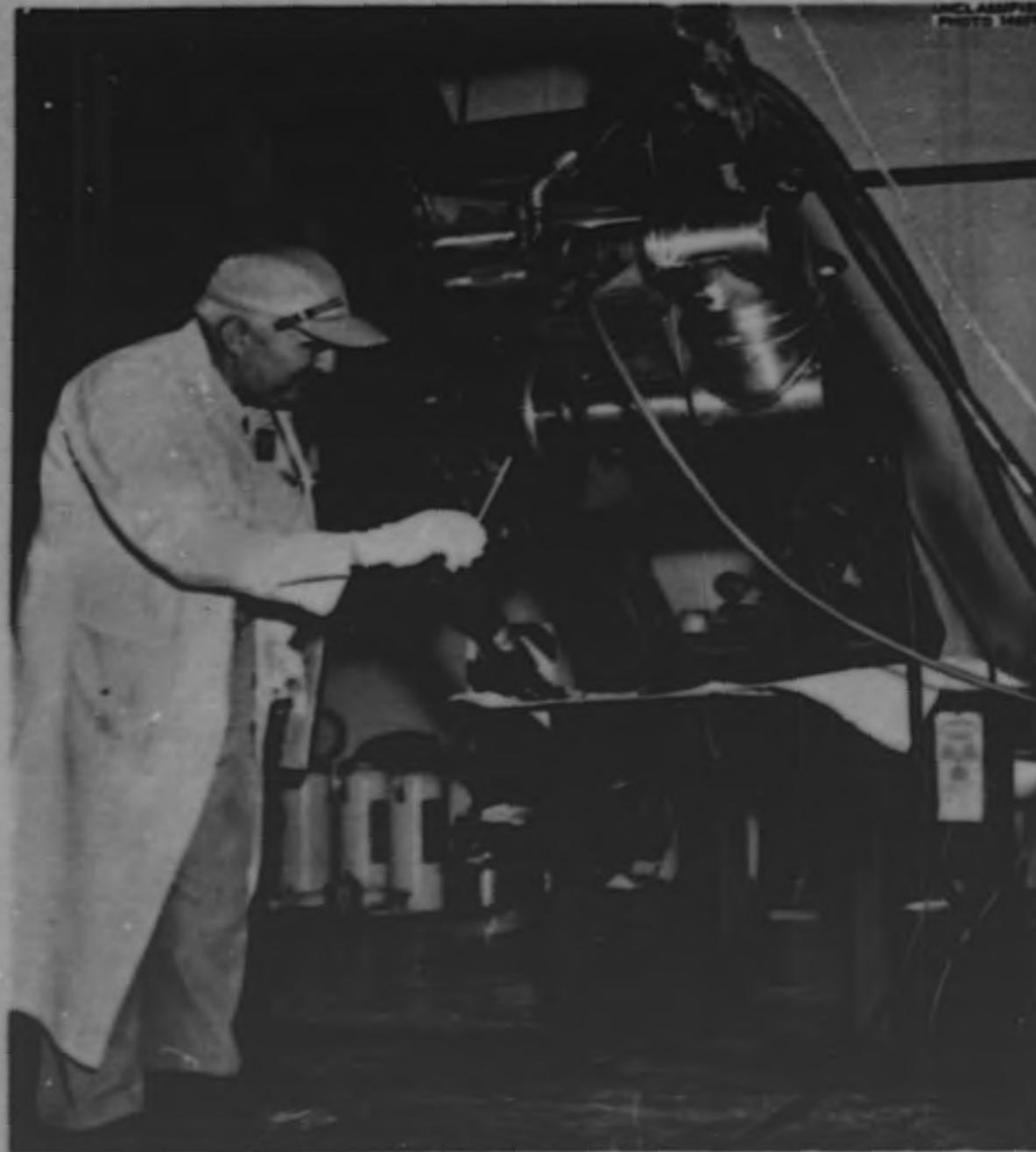
Fig. 11. Cutting Side of Grinder for Dismantling the Reactor.
