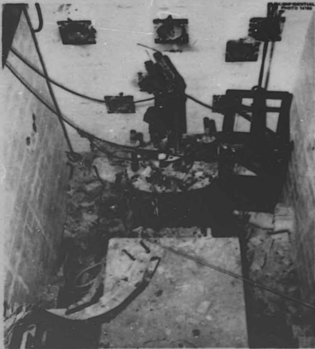
Fig. 9. Gas-Tight Shell Being Removed from Reactor.
