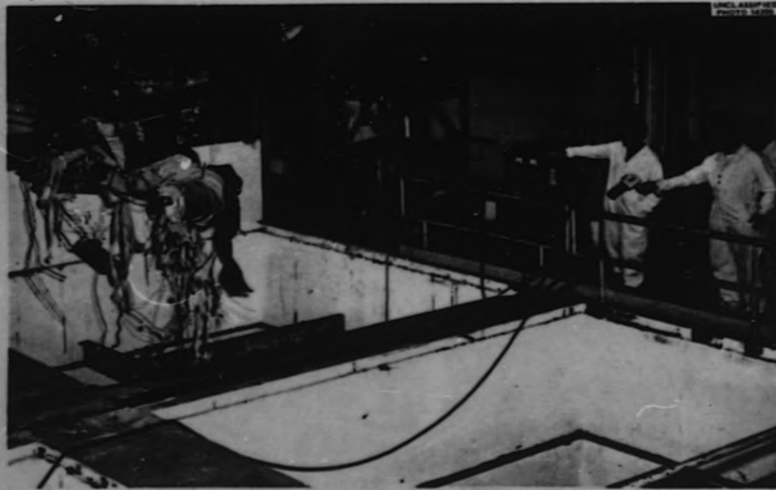
Fig. 7. Main Fuel Pump Being Lifted from Cell.
