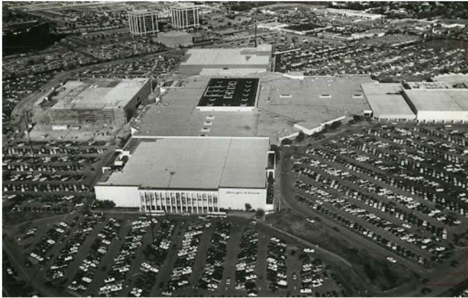
Figure 2.9: Valley View Center Mall, circa 1982. Source: The Dallas Morning News .
