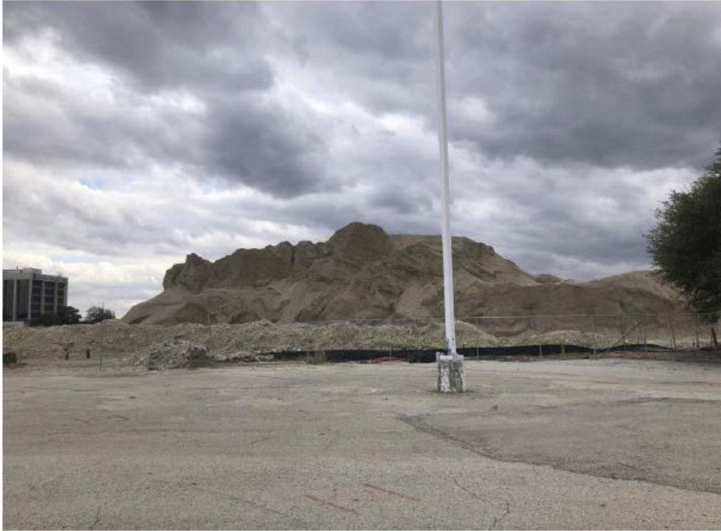
Figure 2.11: Rubble mound during Valley View Center Mall demolition, 2020.
