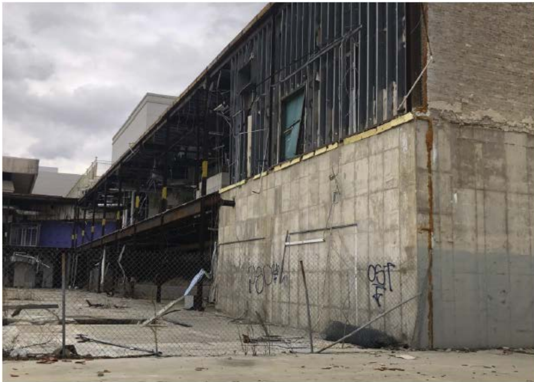
Figure 2.12: Valley View Center Mall mid demolition and graffitied, 2020.
