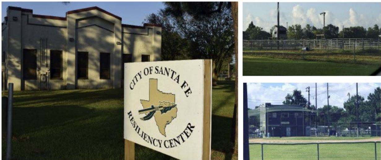
Figure 4.7: Runge Park and the Community Building when Housing the Resiliency Center
