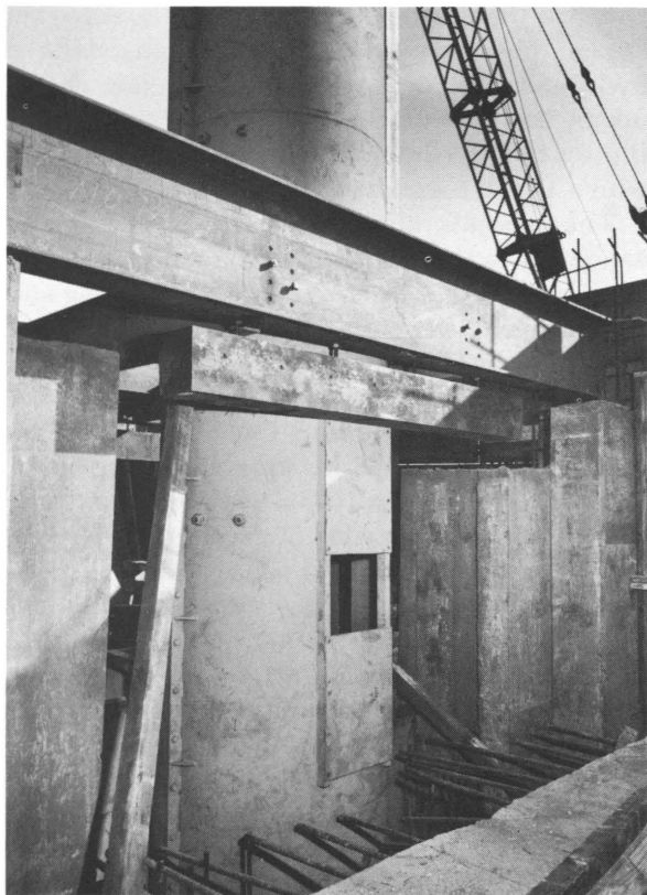
Figure 25. Shutter casing during construction.
