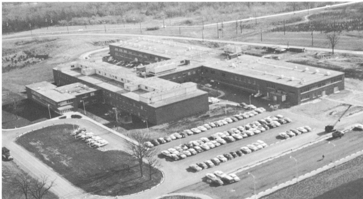
Figure A-1. Fuels Technology Center
