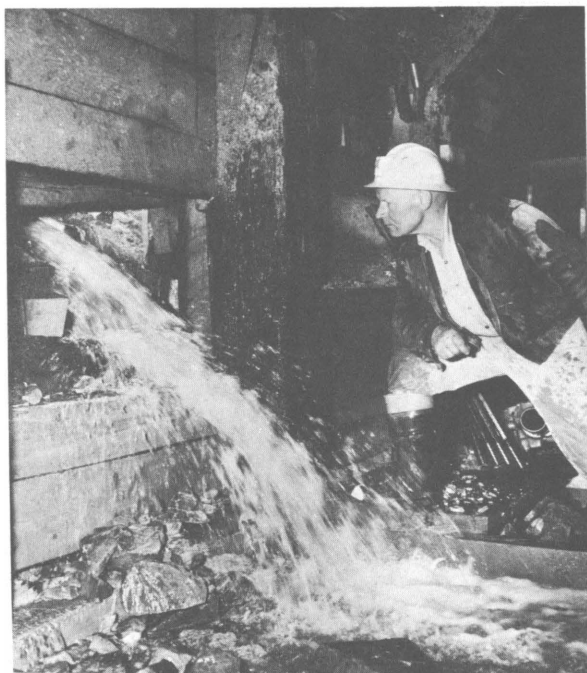
FIGURE 6.—Waterflow Into Mine Drainage Tunnel.
