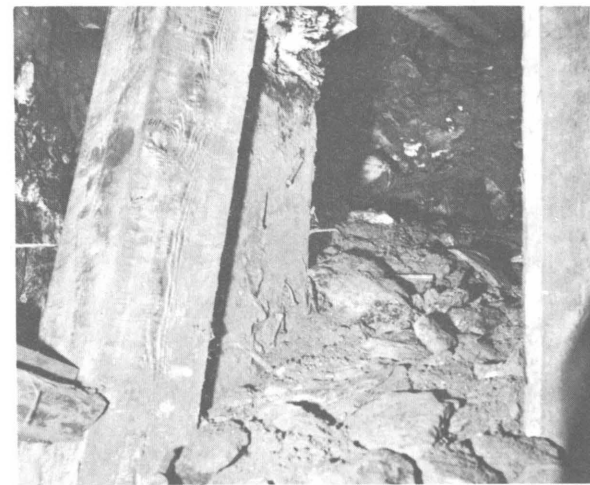
FIGURE 2.—Rock Burst Damage, Galena Mine, Idaho, March 25, 1961.
