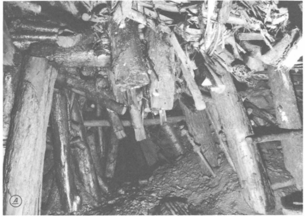
FIGURE 29.—Caved Stopes, Block Caving.
