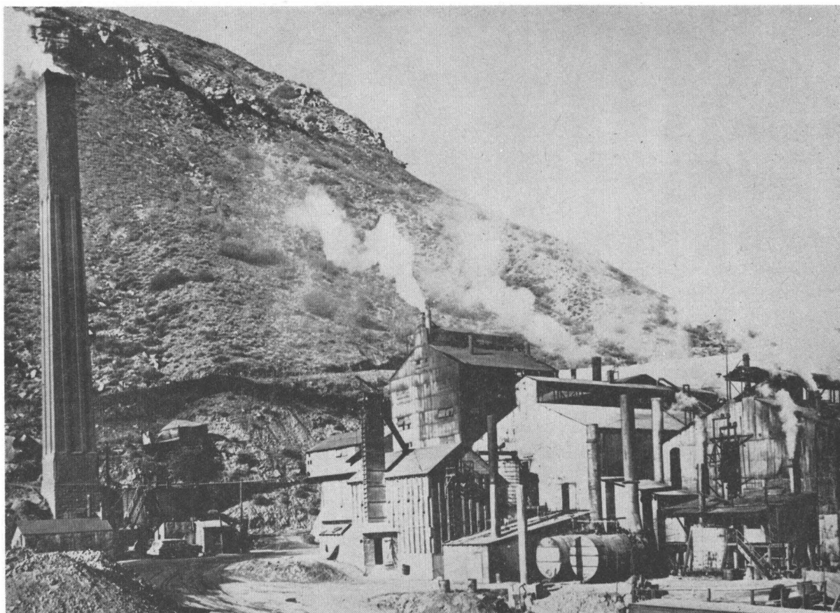
FIGURE 19.—General View of Vanadium Corp. of America's Vanadium-Uranium Mill and Concentrating Plant at Durango, Colo.
