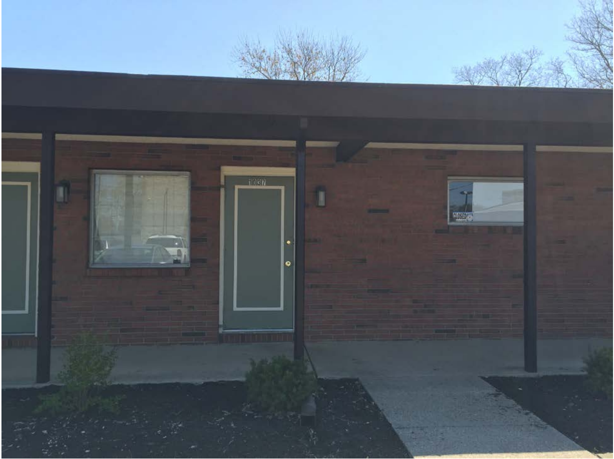
Figure B.8. Photo of Axline's Columbus, Ohio, office.
