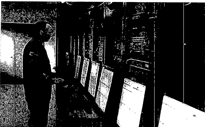
SSL Operations Center
