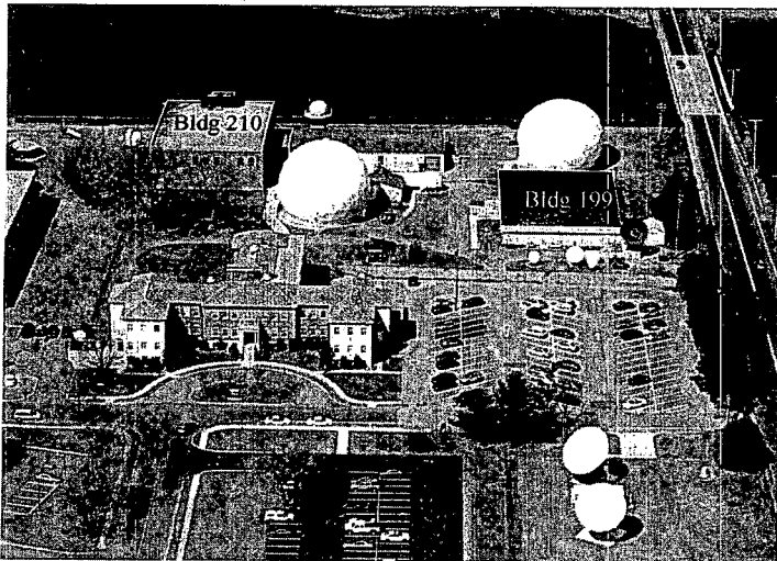
Building 210/199 JSEC Complex
