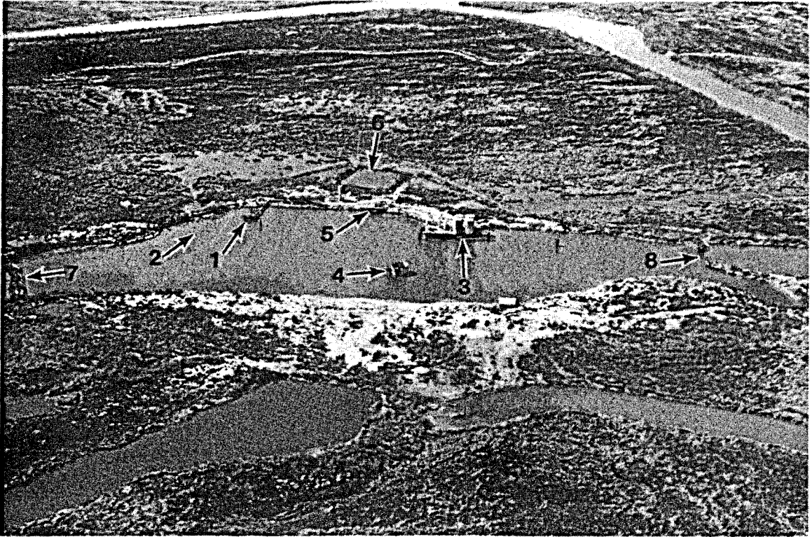
Figure I-5. Aerial view of test-well slip looking to the southwest. Indicated are: the test-well (1), location of disposal well (2), tanks to be removed for conversion of platform to heli-pad (3), plugged well Delcambre #4 (4), platform for condensate storage tank (5), sludge pit (6), dam (7), and bulk heads to be removed (8). White area along edge of slip is unvegetated spoil, the water levels are low and tidal mudflats within marsh are exposed such as to the left and right of the sludge pit.
