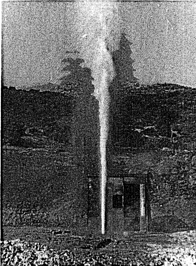
Figure 3. Well G-2 during blowout in 1972.
