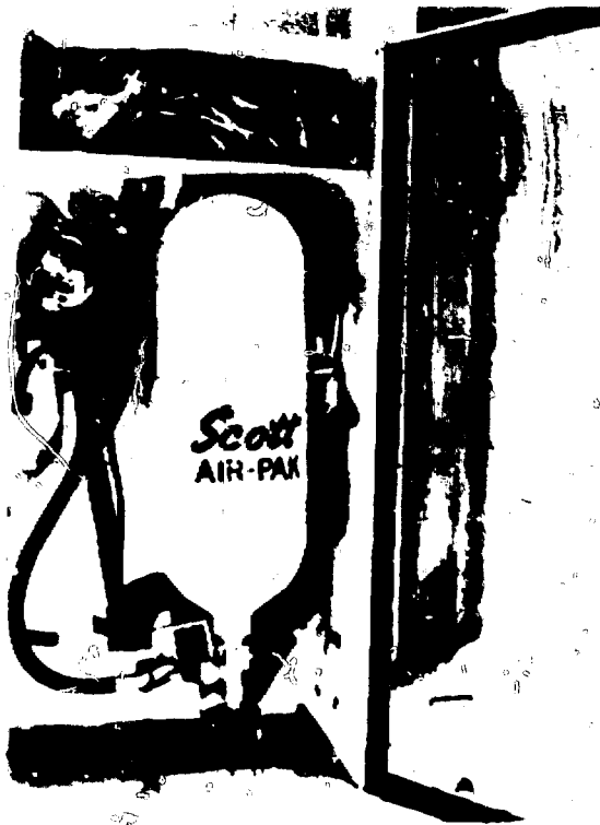
Fig. 9-6. Wall-mounted storage cabinet for a SCBA.
