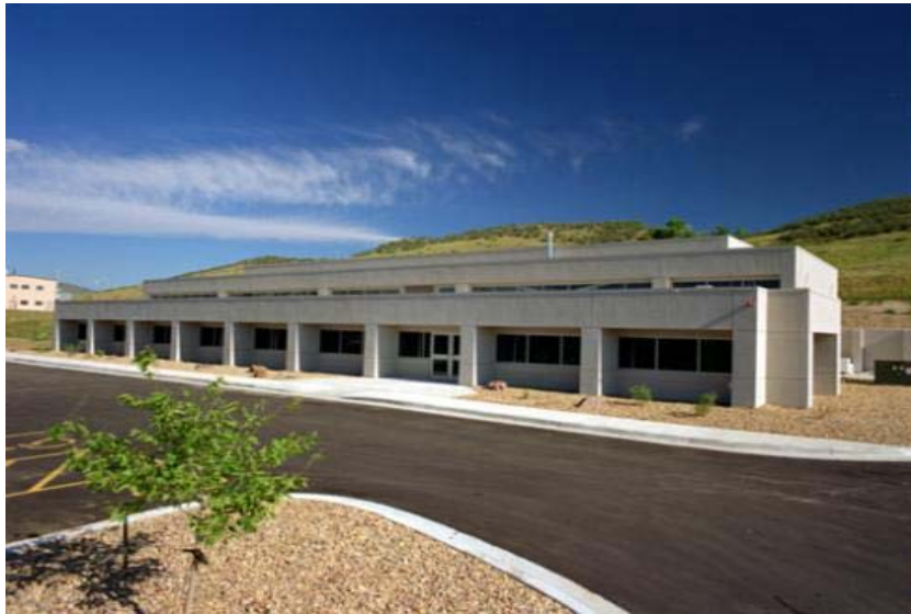
Figure 4-3 Photo of the front of the TTF from the southeast
