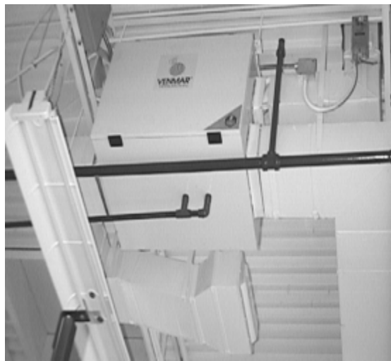
Figure 4-17 Air-to-air heat exchanger removes air from restrooms and kitchen and provides fresh air to building
