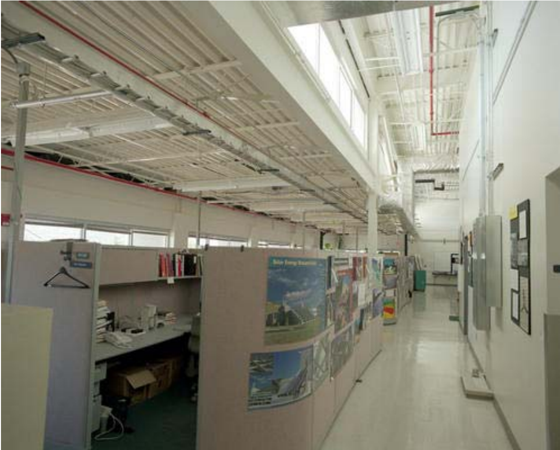
Figure 3-12 Mid-bay clerestory daylight at low-sun angles after installation of blinds
