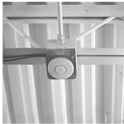
Figure 4-9 EMS-integrated occupancy sensor
