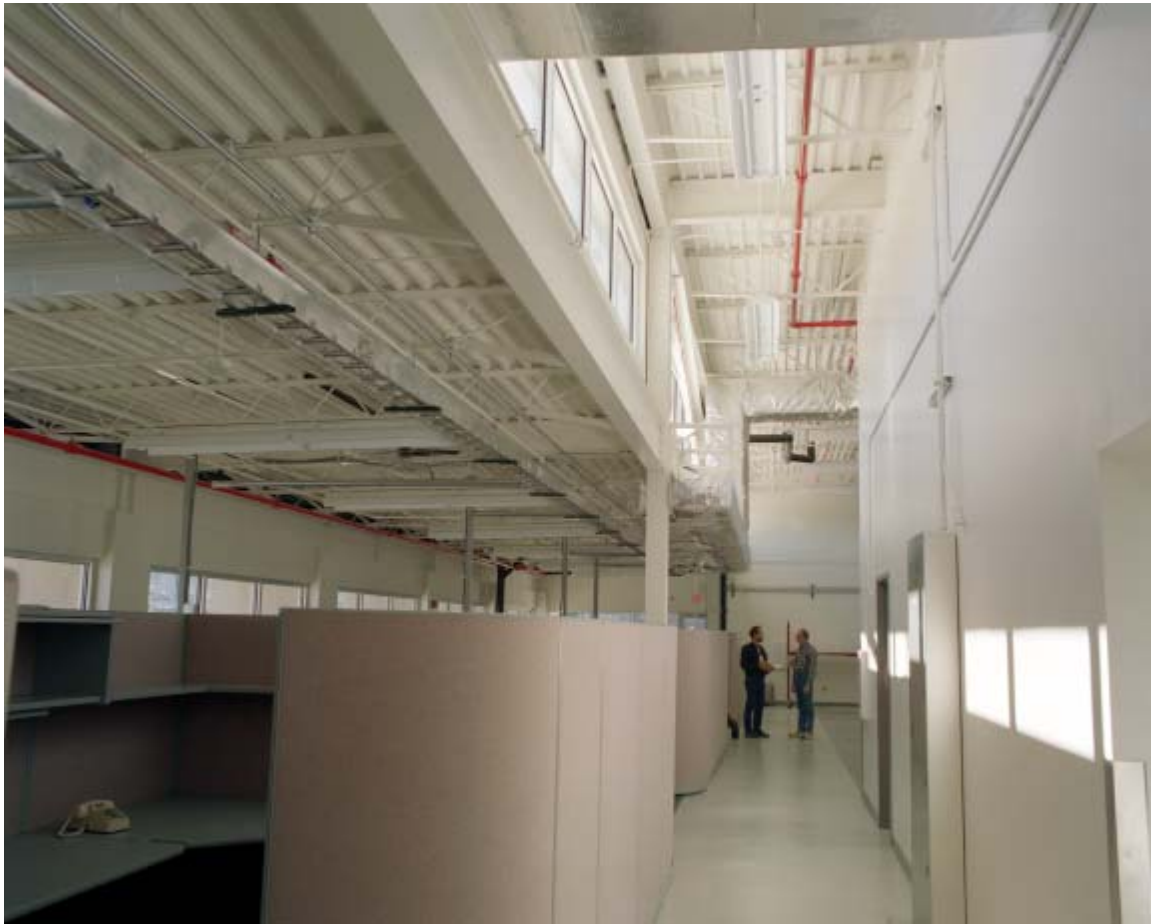
Figure 3-11 Mid-bay clerestory daylight at low-sun angles before installation of blinds
