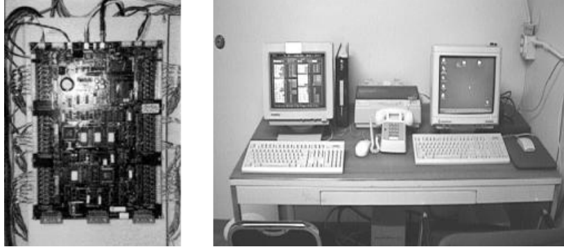
Figure 4-21 EMS input/output panel (left) with PC interface (right)
