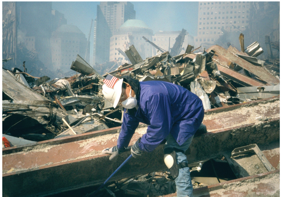
Livermore engineering technologist Mike Newman used a micropower impulse radar sensor attached to an extender to search through rubble at ground zero of the World Trade Center following the September 11, 2001, terrorist attacks.
