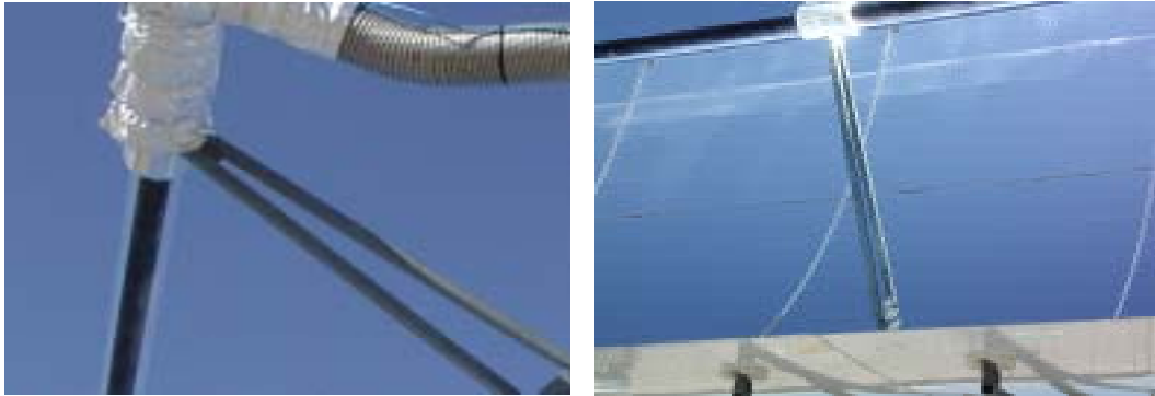
Figure 2.3 Examples of solar trough receiver support brackets
