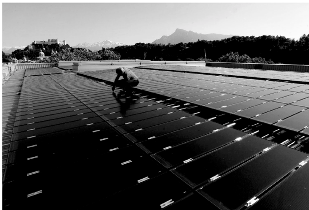
Fig. 9. 40.8-kW thin-film CIGSS PV grid-connected array at Salzburg, Austria.
