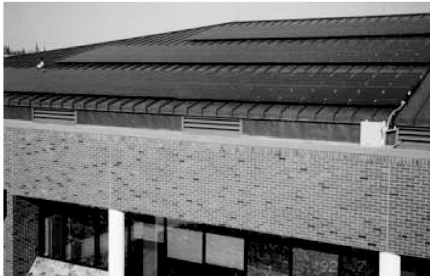
Fig. 8. 10-kW thin-film Apollo CdTe rooftop PV array.
