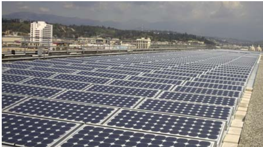
Figure 14: First Gen II Commercial Installation, February 2003
