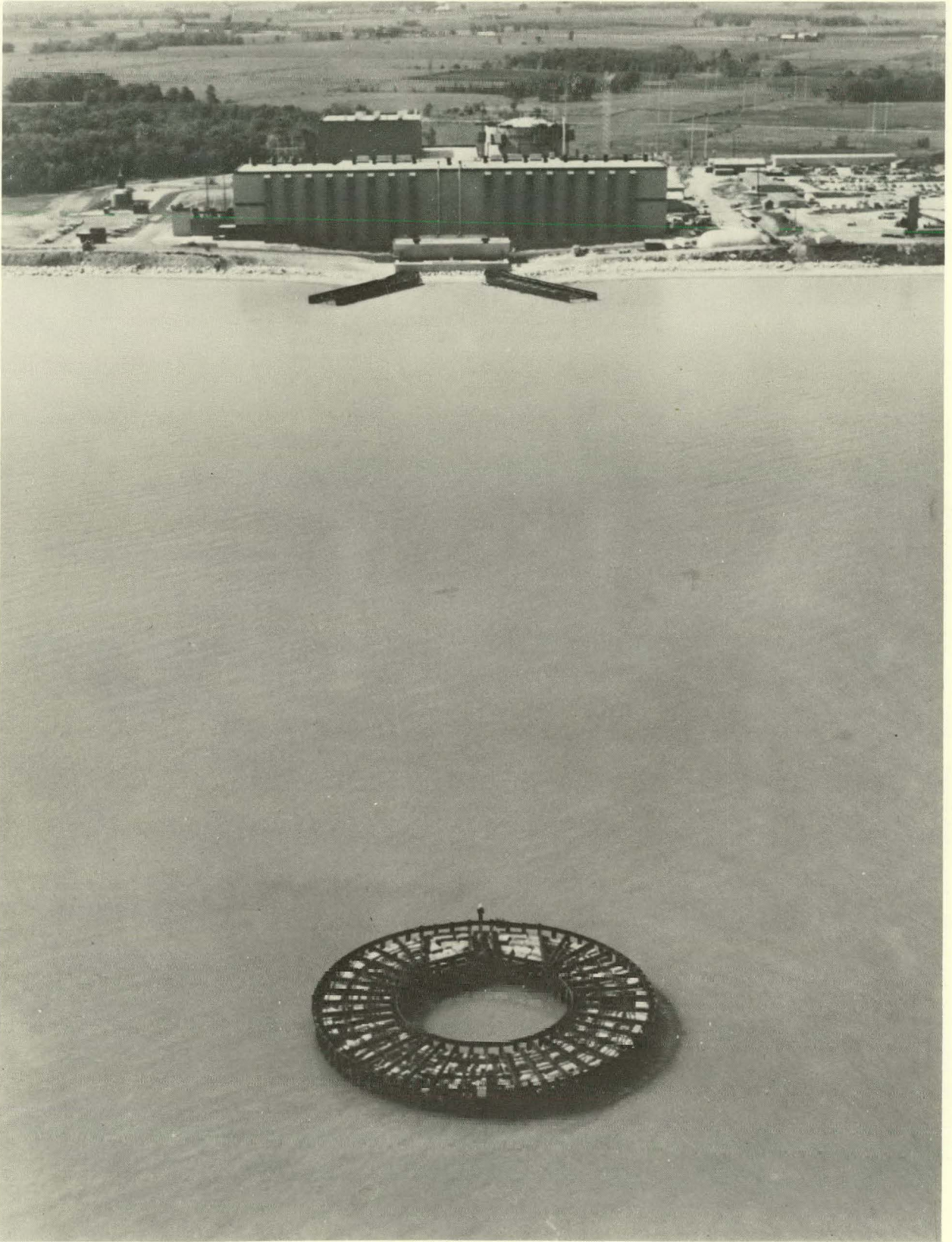
Fig. 1. Aerial View of Plant and Intake Well.
