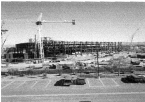
Figure 5. Early LB construction photo
