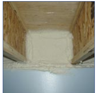
Spray-in foam insulation. Soy-based foams are now available (Photo: Building Science Corporation)
