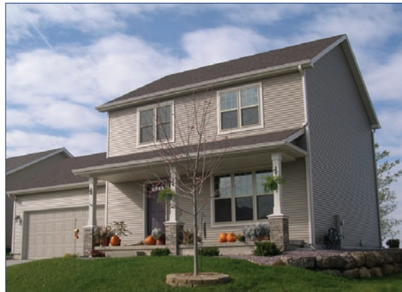
Don Simon Homes (now Veridian Homes) worked with Building America to redesign its most popular floor plan.
