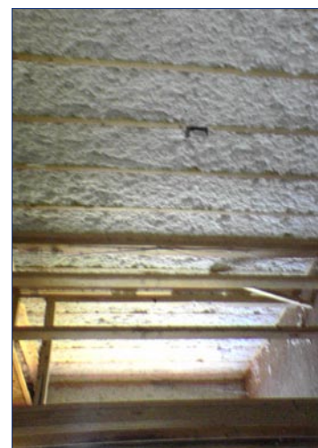
Walls are 2x4 studs insulated with blown-in fiberglass to R-15 plus two inches of extruded polystyrene (R-10).
