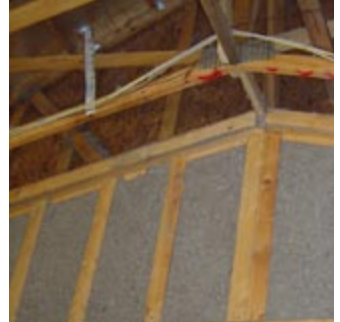
Blown-in wall insulation
