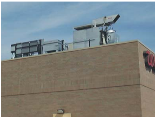
Figure 10. Chesterton site initial and current CHP systems
