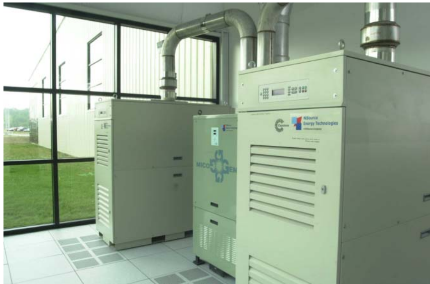
Figure 98. Turbines and heat exchanger
