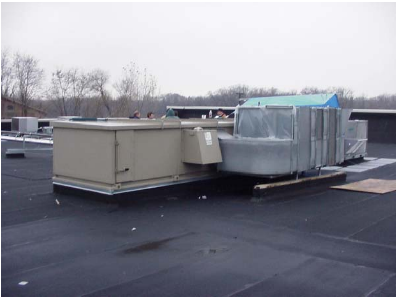
Figure 15. Chesterton site initial and current CHP systems
