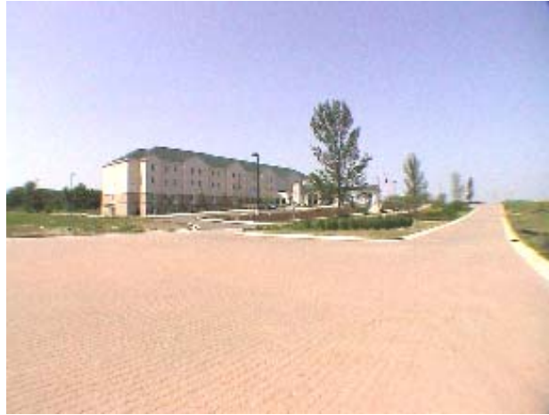
Figure 3: Hotel Test Site
