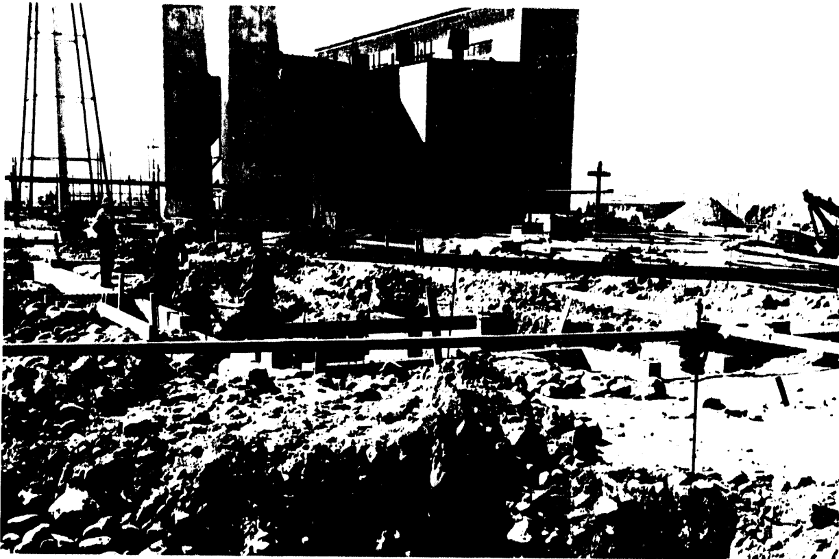
Figure 2-4. The 184-B Power House Under Construction, May 1944.
