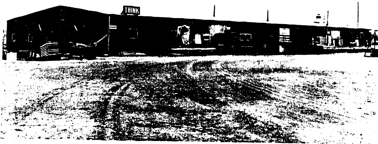
Figure 4-7. The 3722-A Area Shop, Converted From the 300 Area's TC Receiving Warehouse, 1944.
