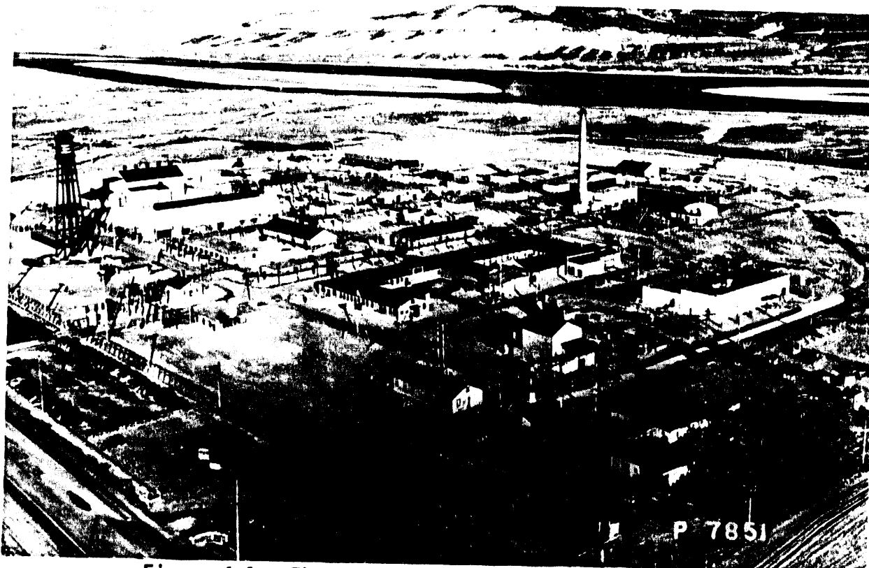
Figure 4-1. The 300 Area, Newly Completed in 1945.
