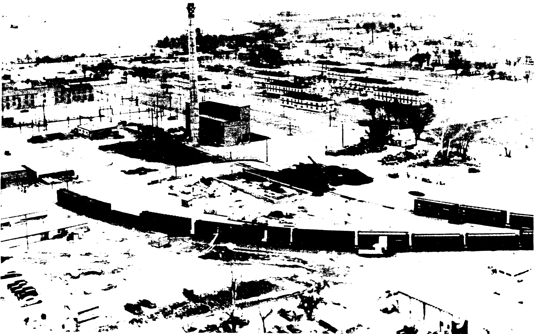
Figure 7-2. The 784 Power House and Its Coal Supply, Richland, 1944.
