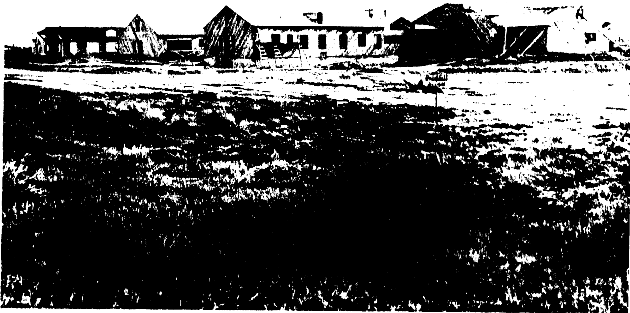
Figure 8-14. The 1118 Richland General Hospital (Later Renamed Kadlec Hospital) Under Construction, February 1944.
