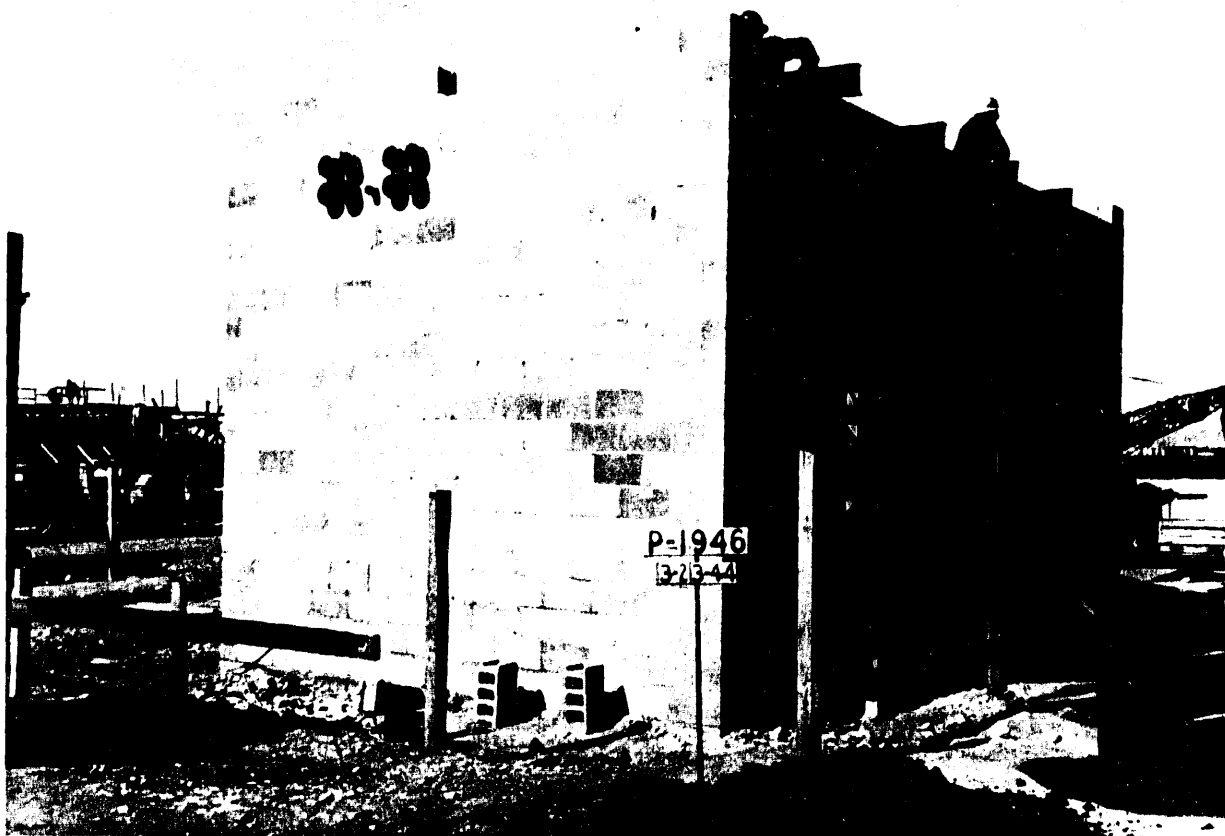
Figure 3-18. The 252-W Secondary Substation Under Construction, March 1944.
