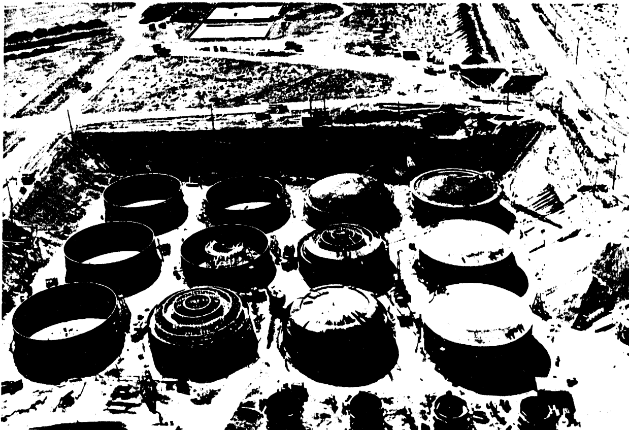
Figure 3-9. Another Original 241-T Tank Farm Under Construction, Mid-1944.
