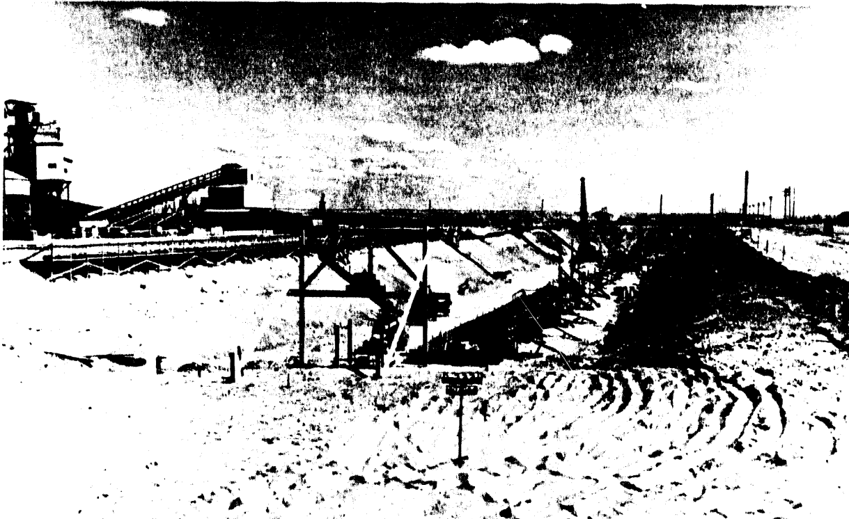
Figure 3-6. The Beginnings of the 221-B Cell Building (B Plant) in April 1944. (The plant began the chemical processing of irradiated fuel rods one year later in April 1945.)
