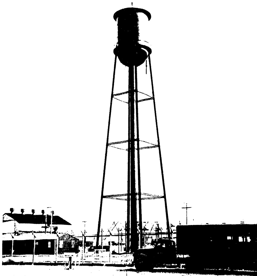
Figure 5-4. Typical Elevated Water Storage Tank at Hanford Engineer Works. (This 3902 Structure held a 75,000-gal reserve for the 3709 Fire Headquarters.)
