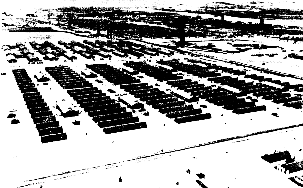
Figure 9-2. The HC-2 Hutments in the Hanford Construction Camp, 1944. (More than 10,000 men, but no women, were housed in such units.)
