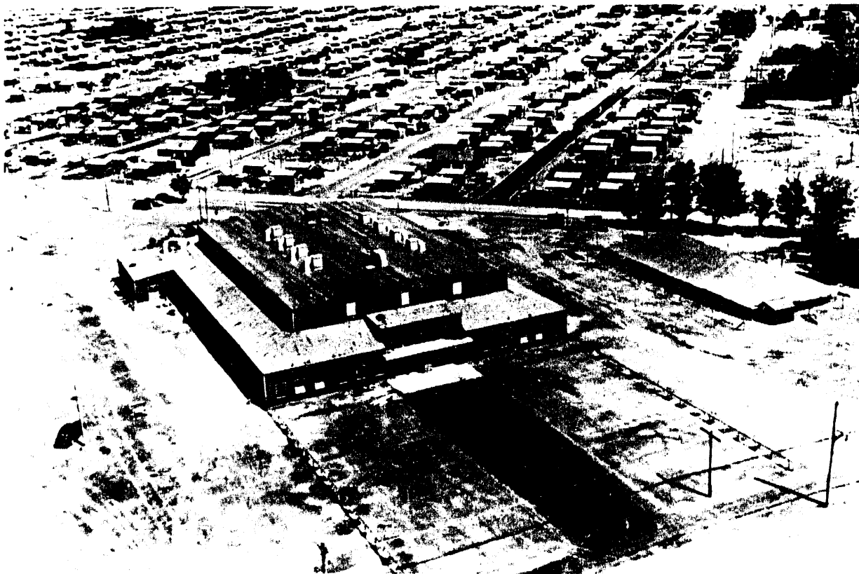
Figure 9-10. The Auditorium and Gymnasium Building (HC-14) Being Completed, July 1944.
