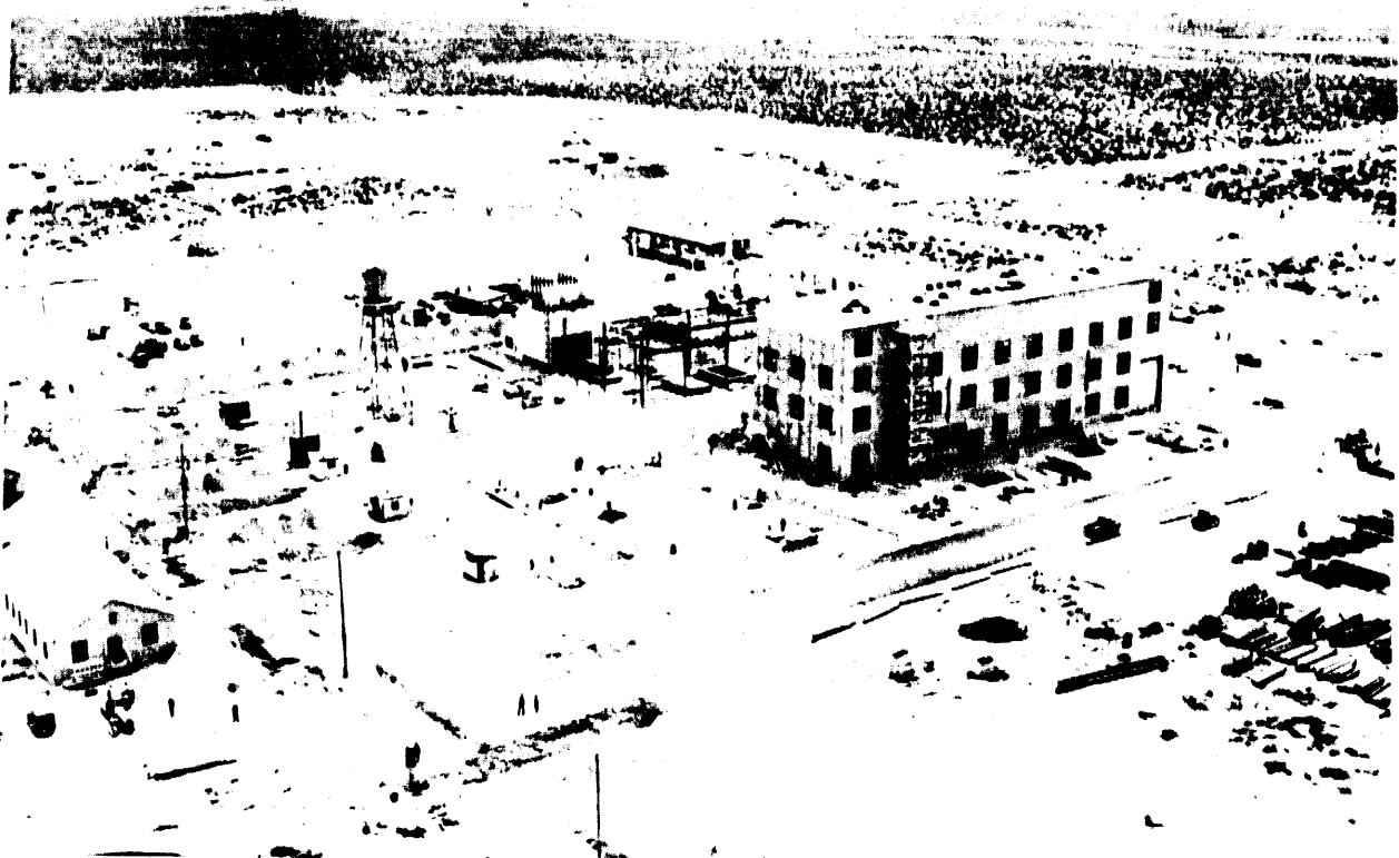
Figure 3-11. The 272-E Area Shop Building Under Construction, Early 1944.
