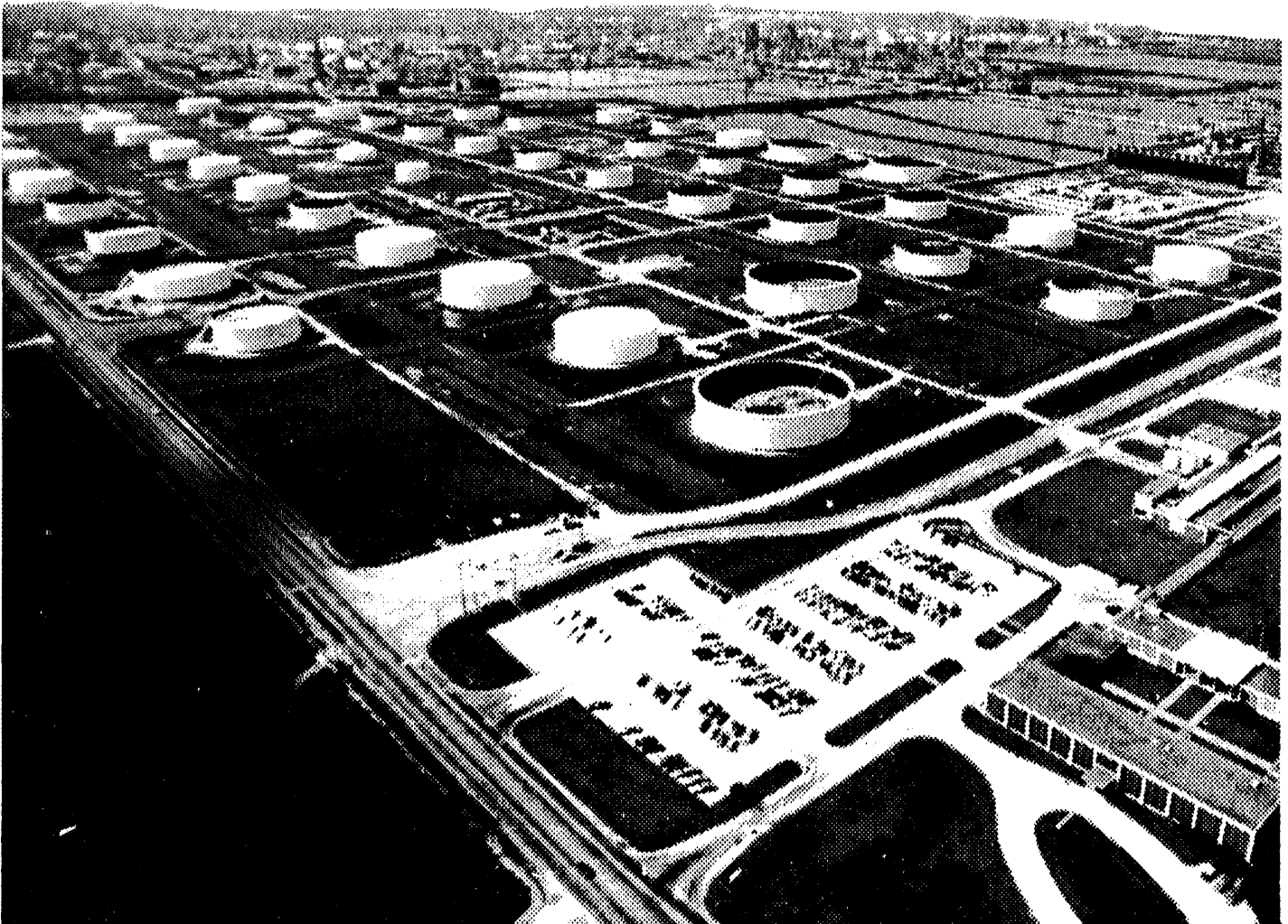
Overall view of a typical bulk terminal facility.
