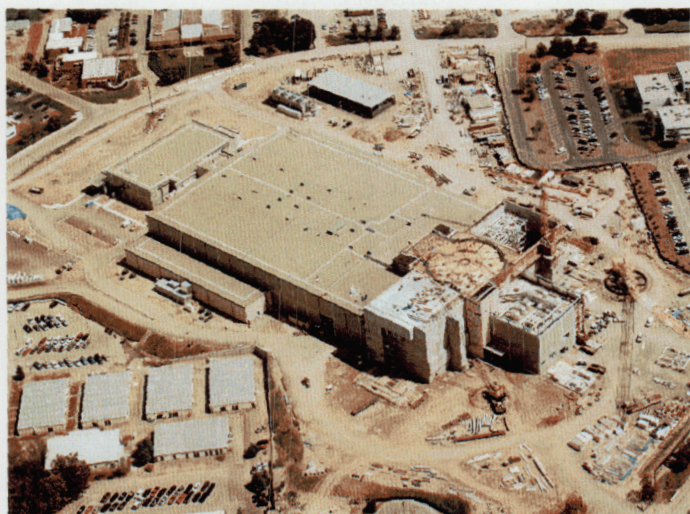
The state of NIF construction early in 2000.
