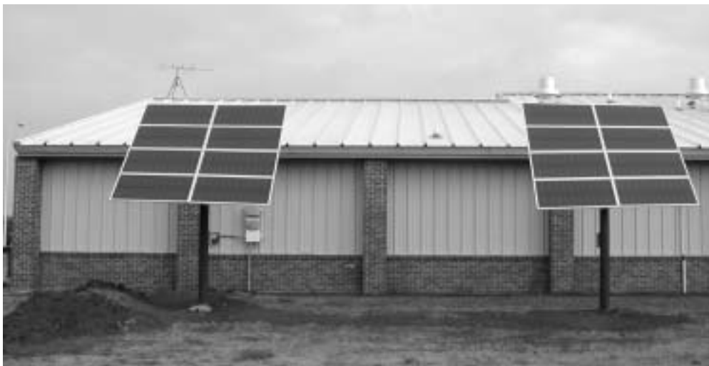
Completed kW PV System, Flandreau Santee Sioux Tribal Clinic
