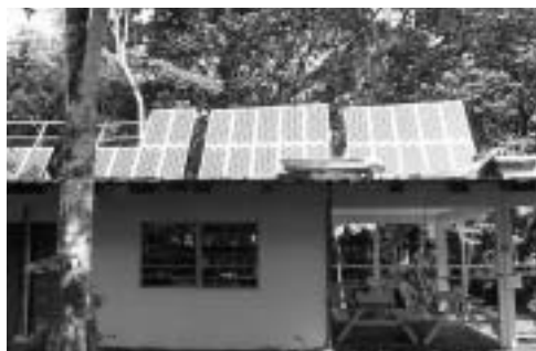
PV system being installed at STRI Republic of Panama
