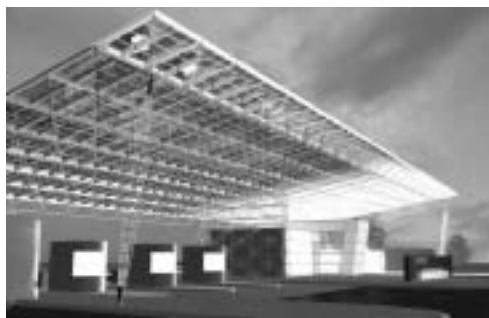
BI PV Canopy for Gatehouse at NASM Steven F. Udvar-Hazy Center
