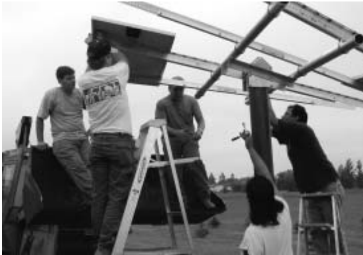
Field instruction in mounting a PV array.
