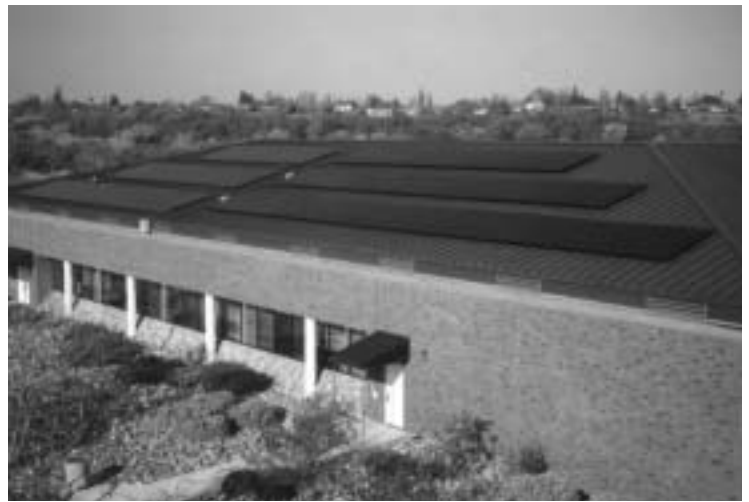
Left Roof: 10 kW BP Solar cadmium telluride ("Apollo") PV System Right Roof: 12 kW Siemens CIS PV System
