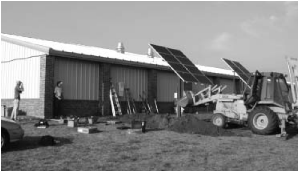
Array installation completed. The next step utility interconnection and clean-up.
