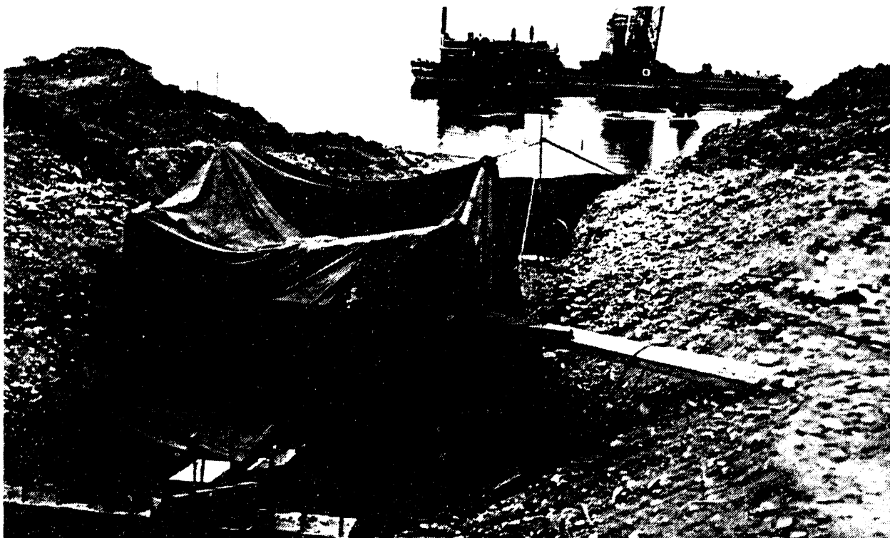
Figure 4-31. Construction of the 190-B Outfall Line, Part of Project CG-558, in December 1954.
