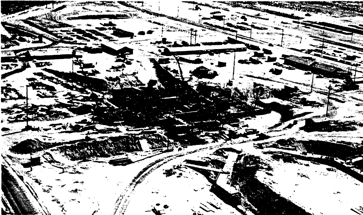
Figure 2-4. 105-C Reactor Building Under Construction, September 1951.
