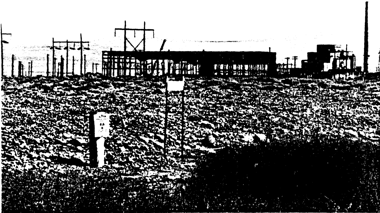
Figure 5-10. 105-B Burial Ground, Looking Northeast (118-B-1).
