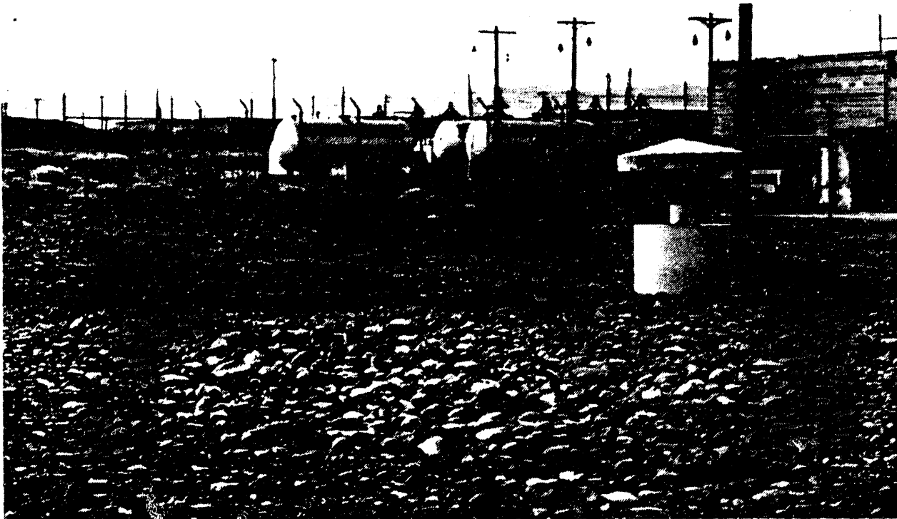
Figure 4-11. Historical Photograph of the 117-B Crib (116-B-12).
