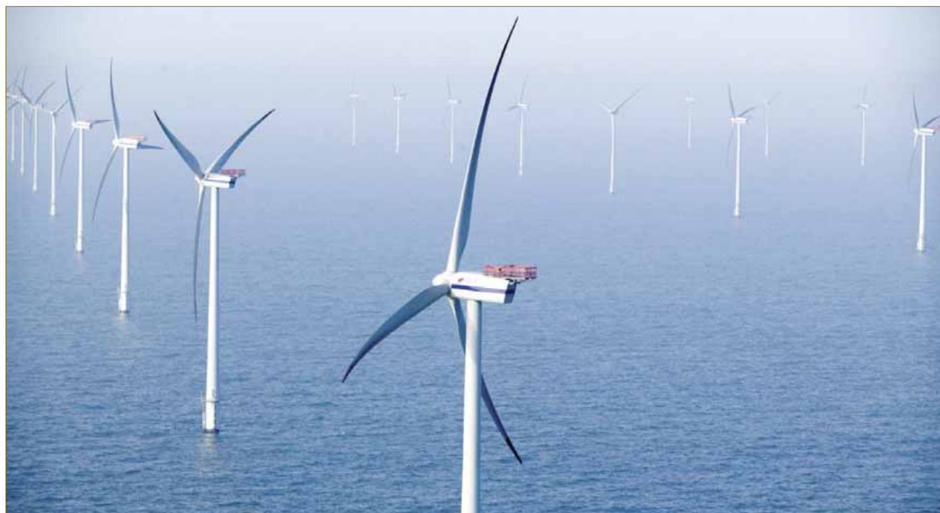
Offshore wind power is a crucial energy source for large cities in coastal locations such as London. 25% of the UK's electricity is to come from offshore wind by 2020, or a total of 29 gigawatts. Higher wind speeds at sea and larger turbines of up to 6 MW offset part of the higher cost of producing electricity offshore. Credit: London Array.
