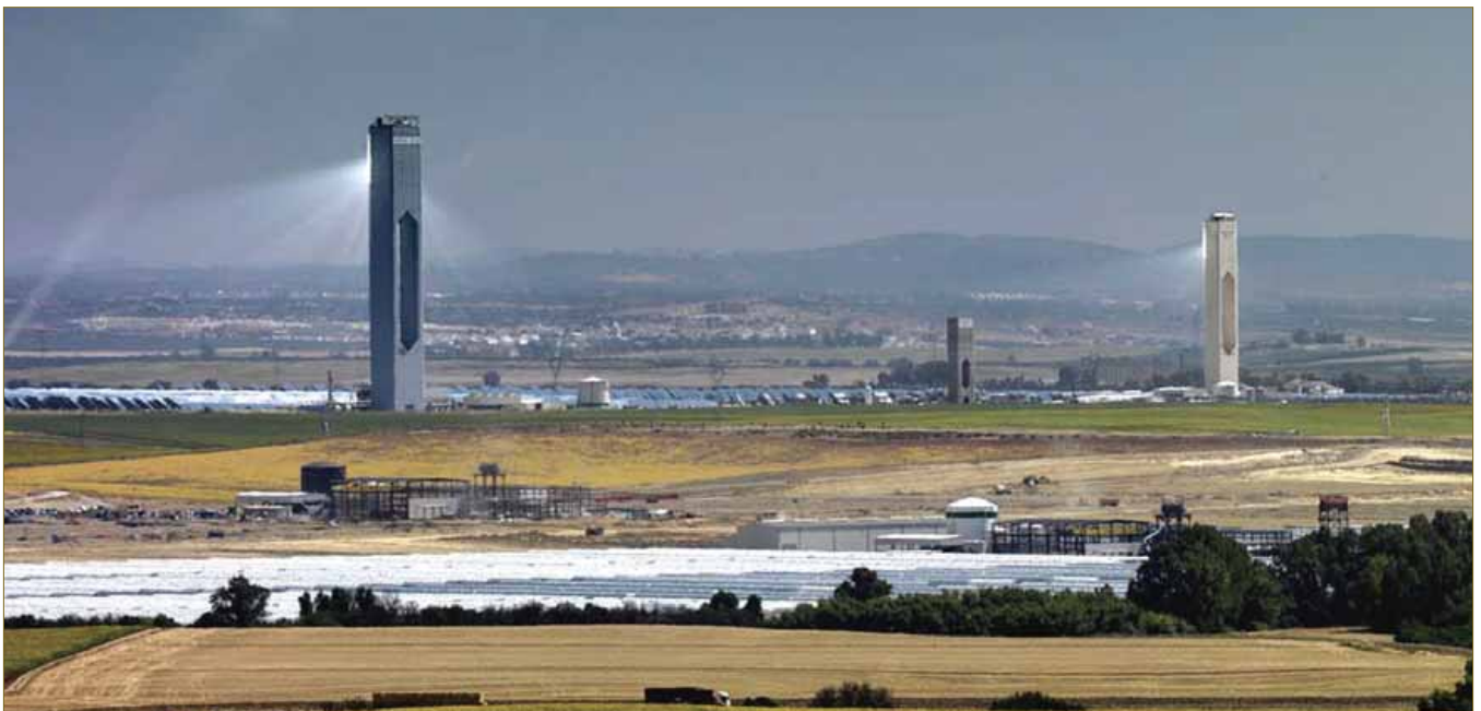
Seville is well on its way to become a city fully powered by solar energy. The solar towers above are about to be joined by several others using the latest solar energy technology which can store heat and supply electricity even after dark. Credit: Abengoa.
