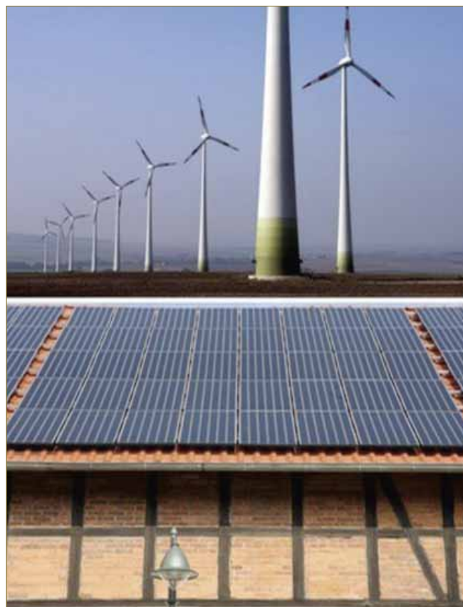
The East German town of Dardesheim combines electricity from PV roofs, wind turbines and biomass burners into a sustainable energy system. Dardesheim is not just self-sufficient but has become a net exporter of electricity to the national grid with considerable financial benefit to the local population. Credit: Dardesheim Tourist Office.
