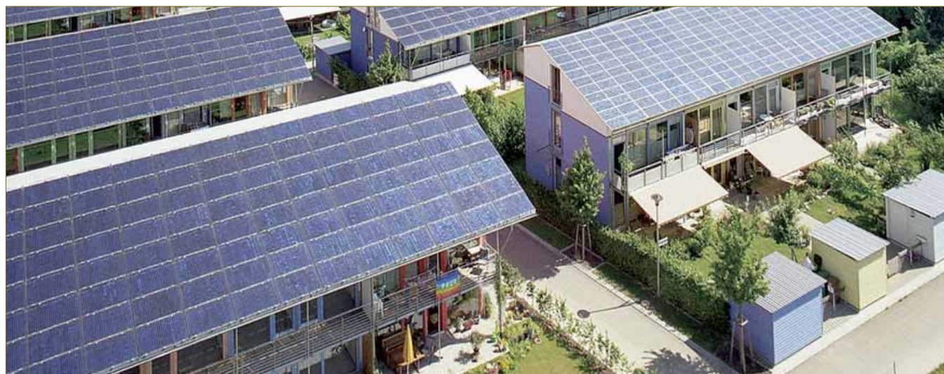
The pioneering 'Solarsiedlung', Freiburg, demonstrates that urban buildings can be designed to produce more energy than they need for their own consumption. Credit: architect Rolf Disch.
