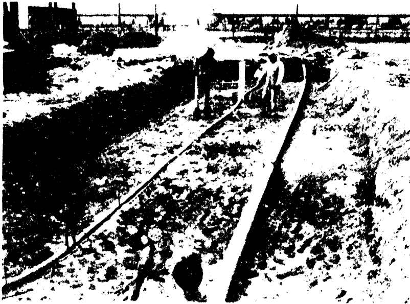
Figure 3. PHOTOGRAPH OF THE LARGE TRENCH LOOKING WEST WITH THE 2-, 4-, AND 6-INCH PIPE
