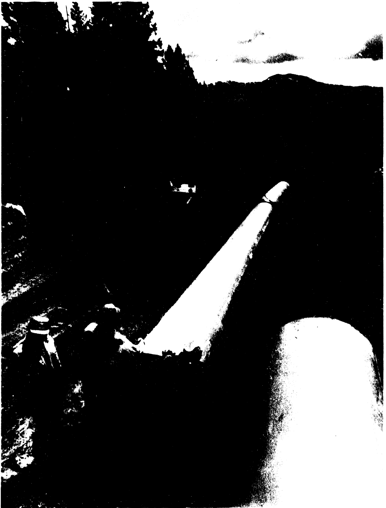
Large pipelines bring natural gas from supply areas to local distribution companies.
