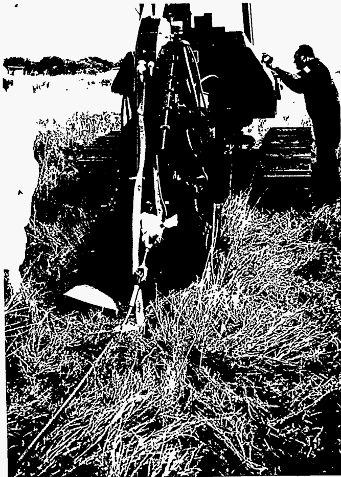
a) Wire rope pulling cable, break link, and load cell attached to HT 100 tractor.
