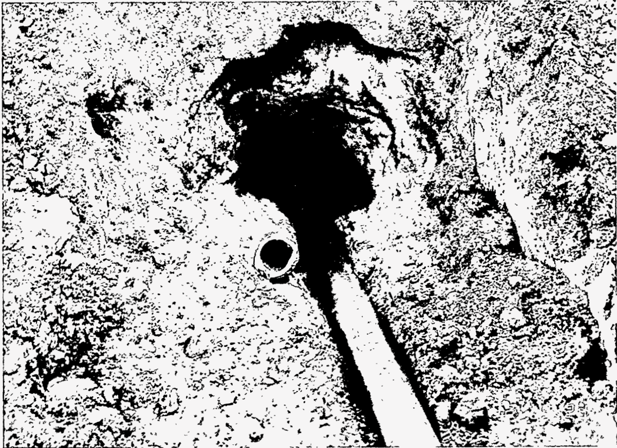
Figure 13. Teflon® casing remnant and new fiberglass casing at SRS.
