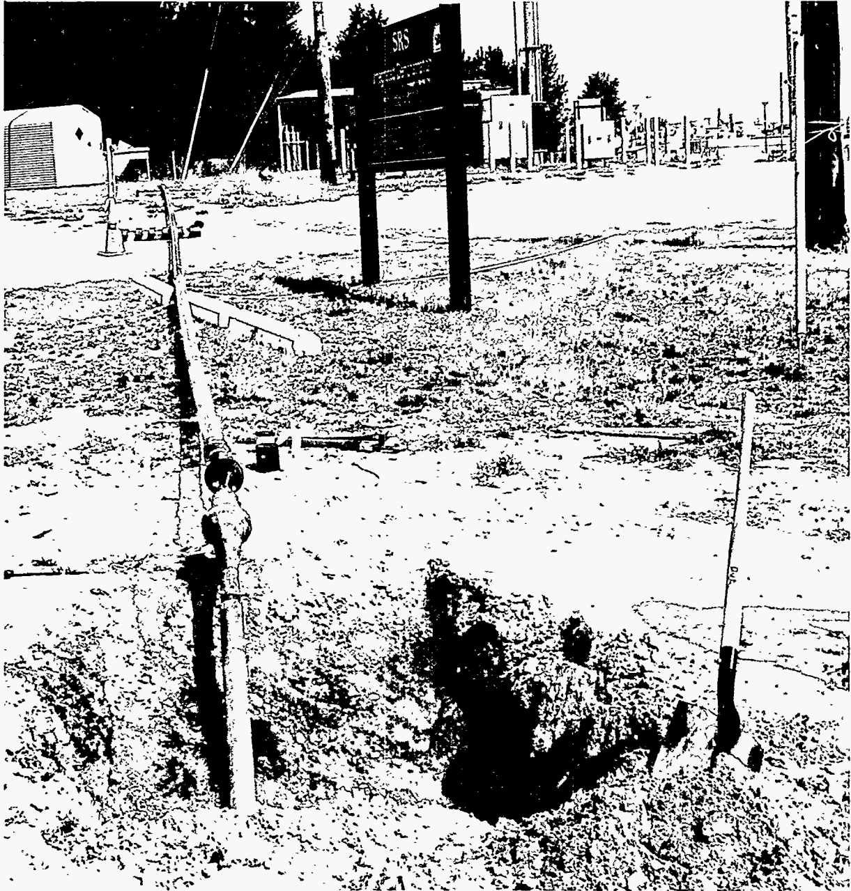
Figure 12. Casing pullback at SRS.
