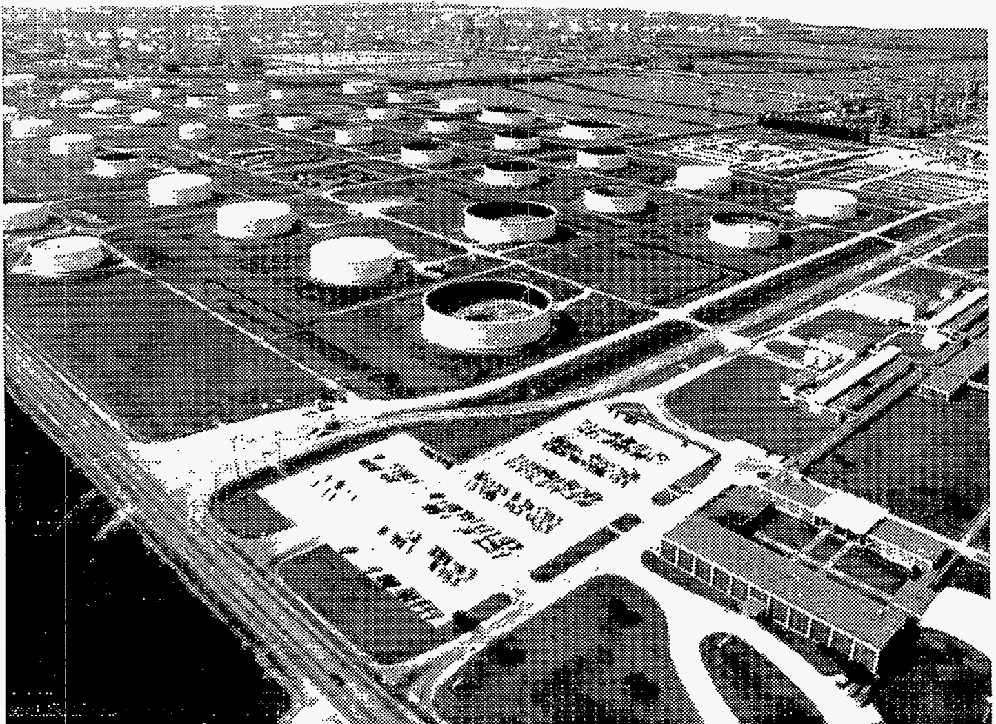
Overall view of a typical bulk terminal facility.
