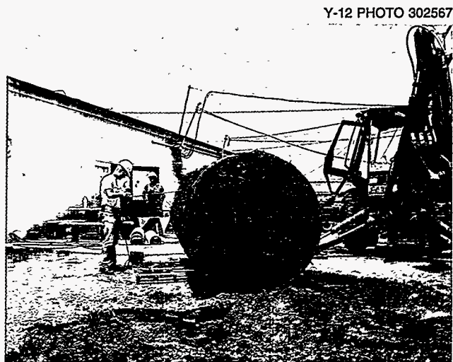
Fig. 3.3. Tank 2395-U, formerly used to store fuel oil, was removed from the Y-12 Plant in June 1993.
