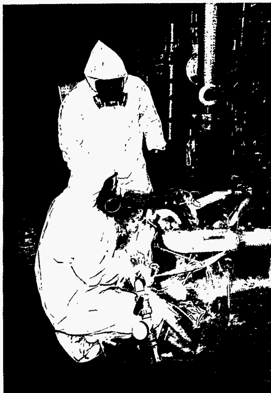
Fig. 3.4. Technicians work on piping covered with asbestos-containing material.
