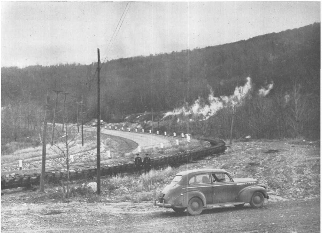
FIGURE 7.—Semicircular Wooden-Stave Flume in Area Complicated by Subsidence and a Mine Fire.
