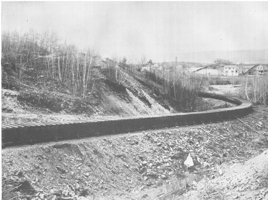
FIGURE 8.—96-Inch, Semicircular, Creosoted, Wooden-Stave Flume.
