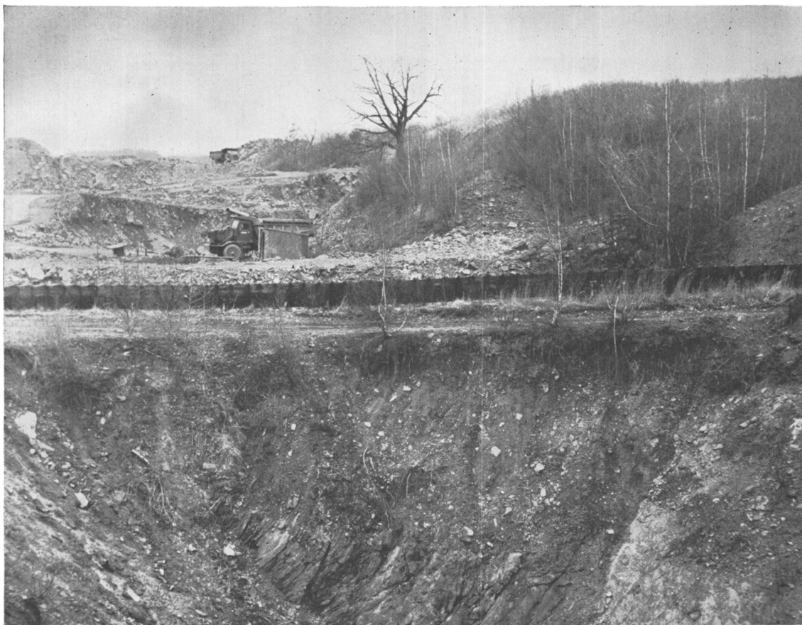
FIGURE 5.—Semicircular Wooden-Stave Flume in Stripping Area.
