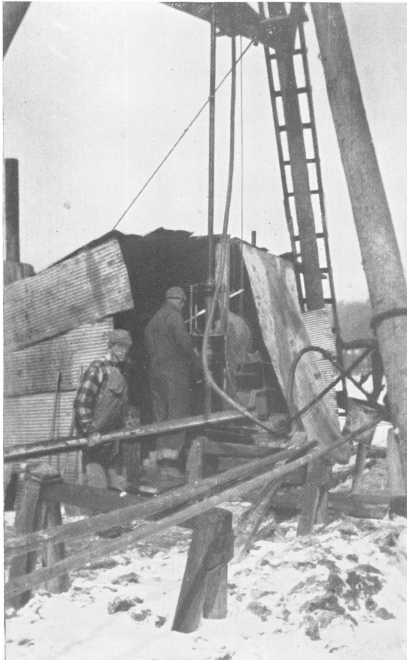
FIGURE 4.—DIAMOND DRILL AT HOLE 38-CB.
