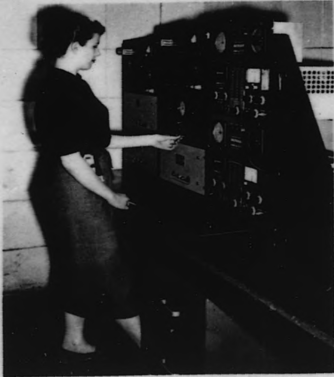
FIGURE 6 UNIT IN OPERATION
